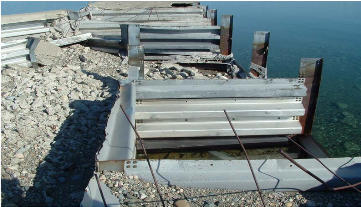
Photo 1: Storms causing waves on Iliamna Lake have caused extensive damage to both the dock and mooring vessels, photo courtesy of Alaska District Corps of Engineers, 2005.
