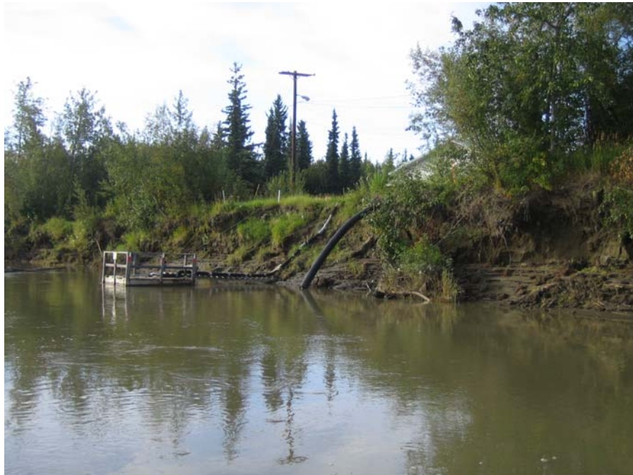
Photo 3: City water intake building to riverbank 20 feet and Cap'n Snow Building to river bank 96 feet. June 11, 2007.
