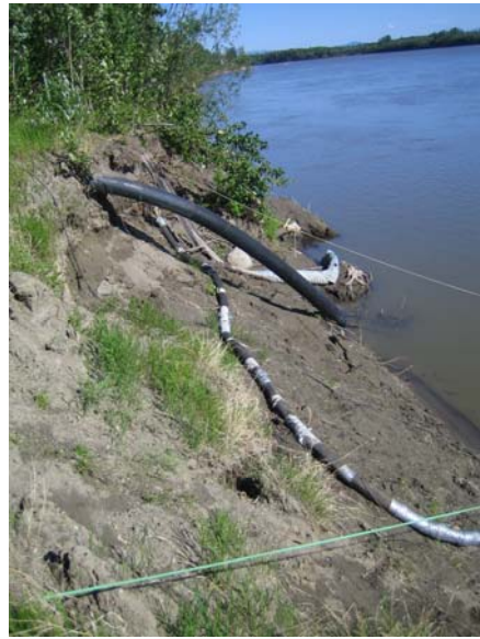
Photo 2: City water intake lines. June 2007.
