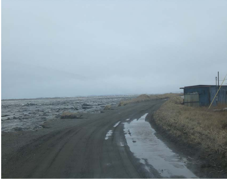
Photo 1: Pilot Point Road along Ugashik Bay leading to the bulkhead dock is threatened by erosion, April 2008.
