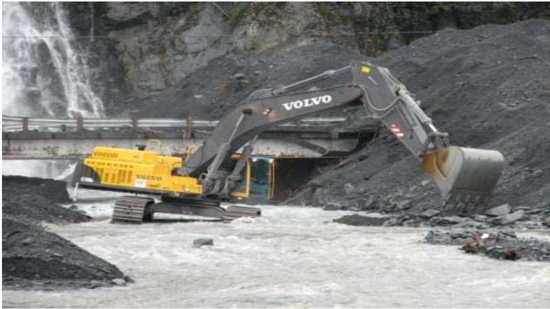
Photo 1: Lowell Creek tunnel outfall being cleared after the October 2006 flood buried the bridge blocking Lowell Point Road, October 2006.
