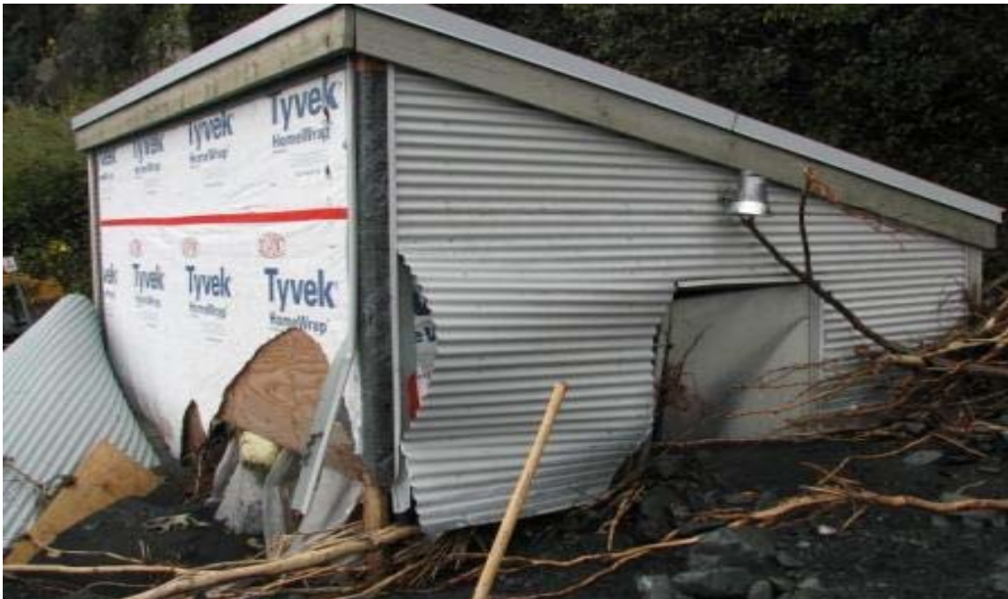
Photo 2: Alaska Sea Life Center outbuilding debris damage from Lowell Tunnel flooding, October 2006.
