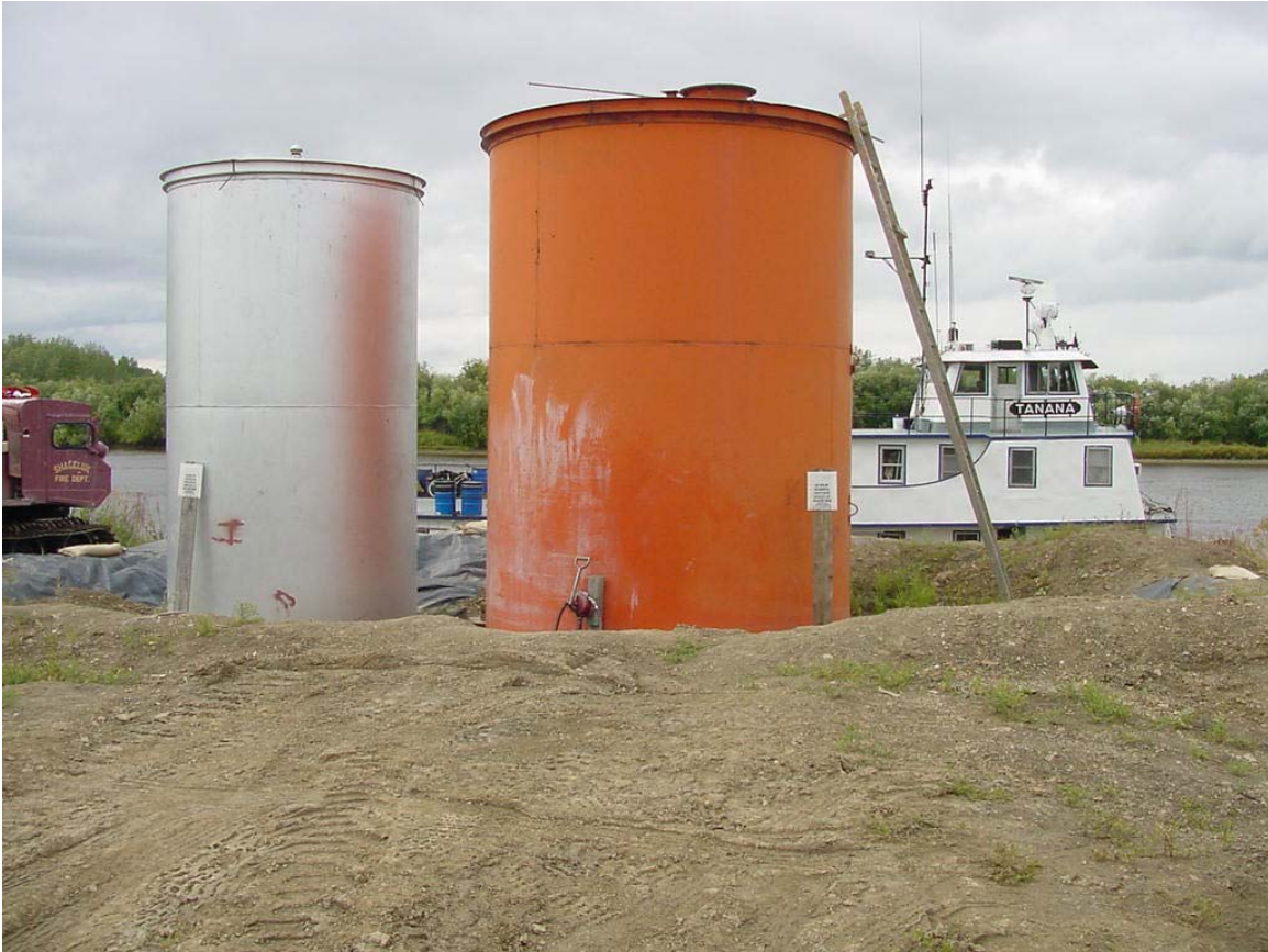
Photo 1: Shageluk city tank farm with fuel barge docked on Innoko River in background. Photo courtesy DEC.
