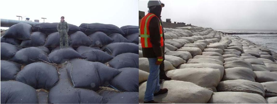
**Figure 13: Photos August 2000 (Left) West Dock 4 cubic yard sandbag revetment. Constructed in 1993, no maintenance has been performed. Lower strength polypropylene bags, tensile strength 500 lbs per inch. (Right) West Dock 4 CY revetment constructed in 2003. These bags use a stronger 1100 lbs per inch polyester fabric. Coastal Frontiers is currently extending this revetment around the end of the West Dock Causeway.**
