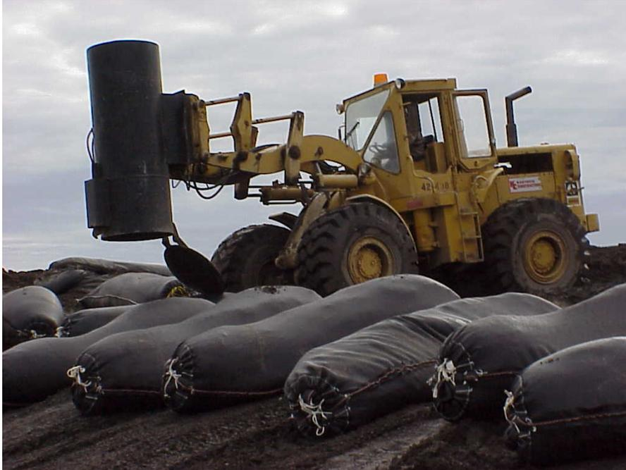
**Figure 22 Steel pipe modified to transport large (4 CY) sandbags.**
