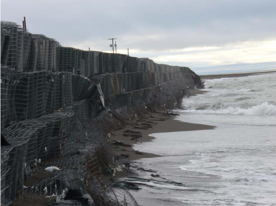
**Figure 1 Failed shoreline project several months after completion of construction.**
