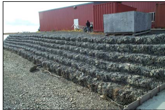
Typical rock filled gabion bank protection
