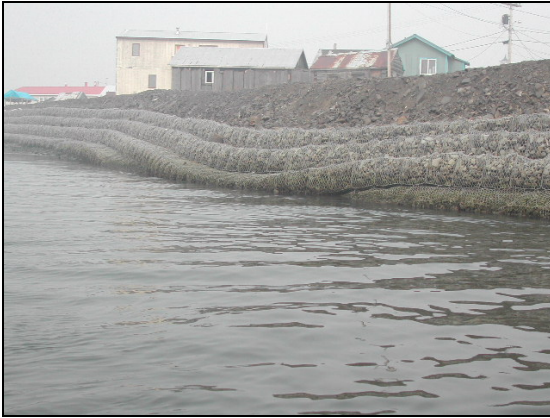
Sagging Gabion Wall
