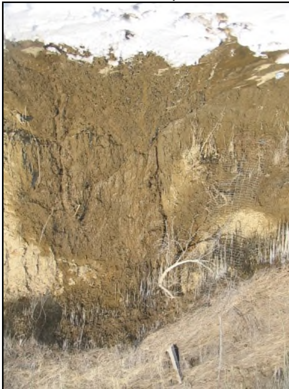
Erosion control fabric and debris
