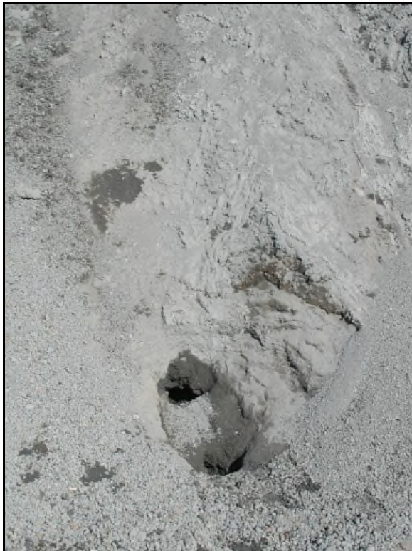
Piping holes near toe
