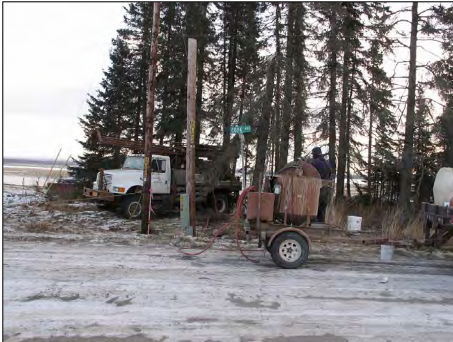
b. Grouting at Group 2 borings. November, 2006.
