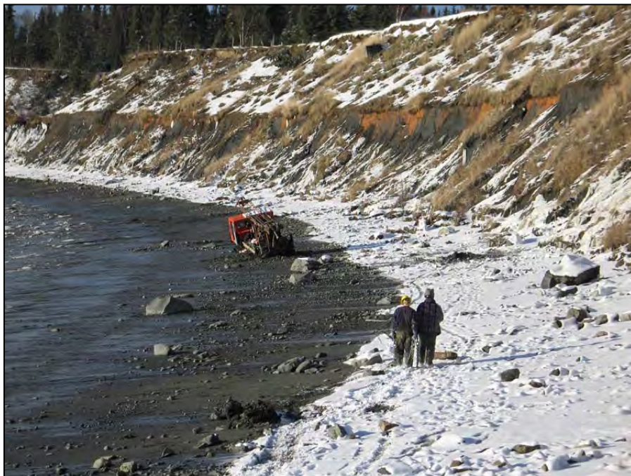
b. Drill stuck in mud near Senior Center. The soft mud made it difficult to use tracked equipment on tide flats. November, 2006.
