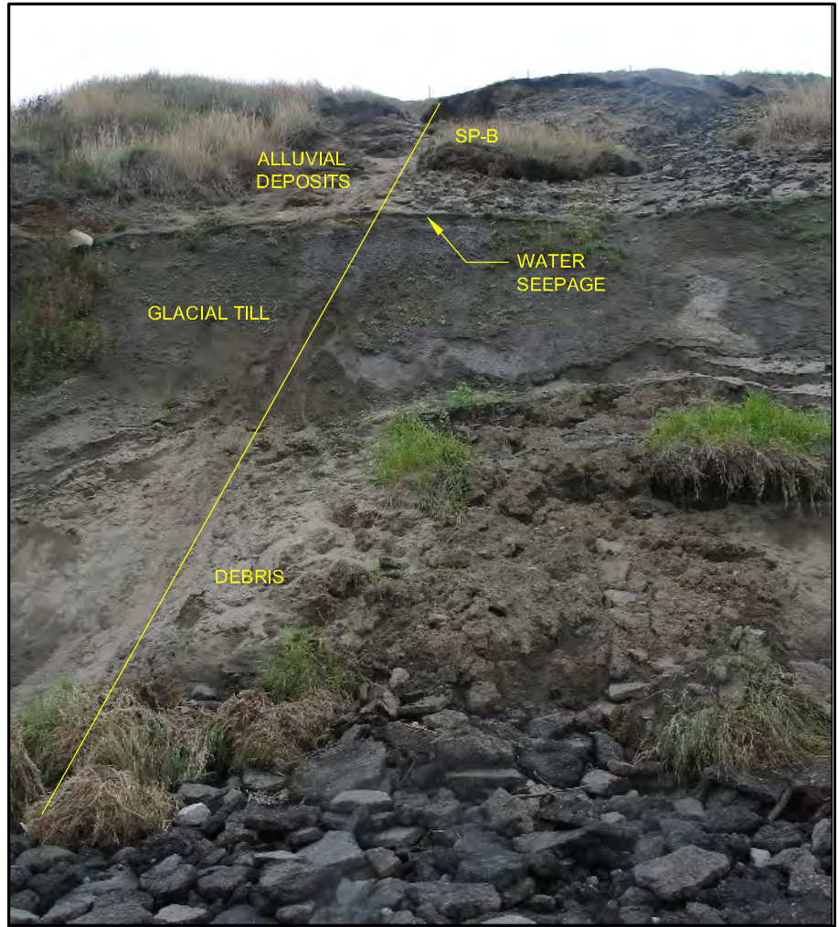
LOOKING NORTH AT SP-B. THE SLABS AT THE BASE OF THE SLOPE CONSIST OF ASPHALT. 10 OCT. 2006
