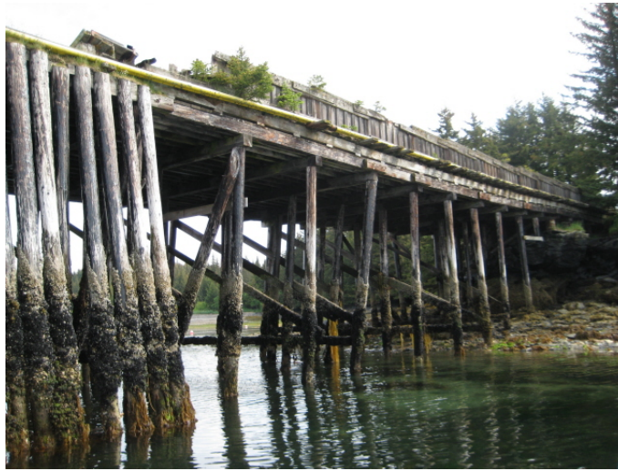
Figure D-7. View showing misaligned pile under causeway
