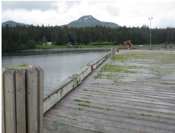
Figure D-11. Typical dock surface with vegetative growth
