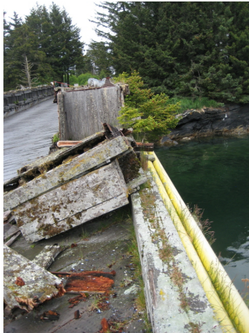
Figure D-12. Decaying live crab pots, fuel lines, and vegetative growth including trees
