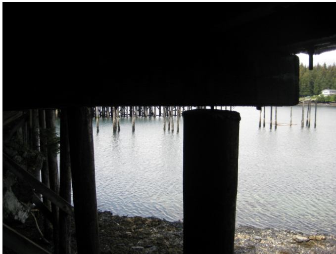
Figure D-2. Gap between pile and dock
