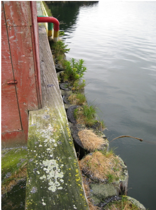
Figure D-1. Vegetation growing atop pile ends
