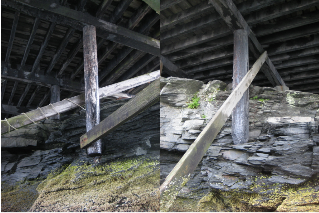
Figure D-3. Unbraced piles on bedrock
