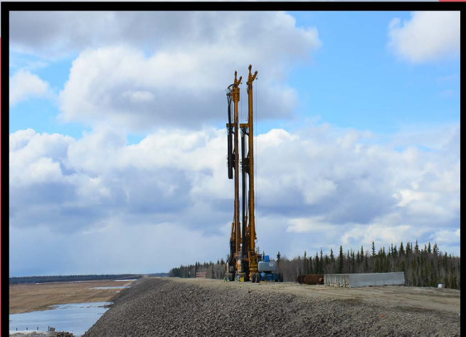
Construction on the Moose Creek Dam Modification Project began May 12, 2022
