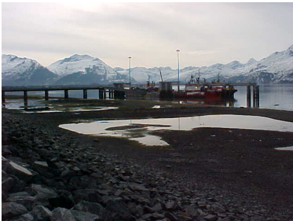
Photograph 3: Eastward view intertidal area of West Site. SERVS Dock in background.
