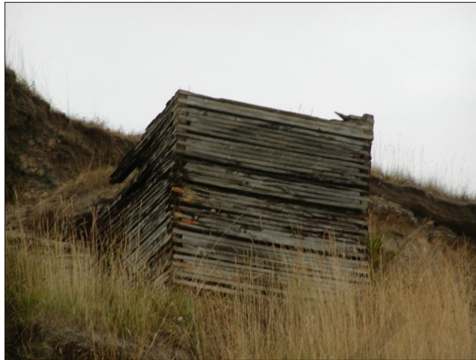
Figure 10. Remnants of unidentified structure number 4
