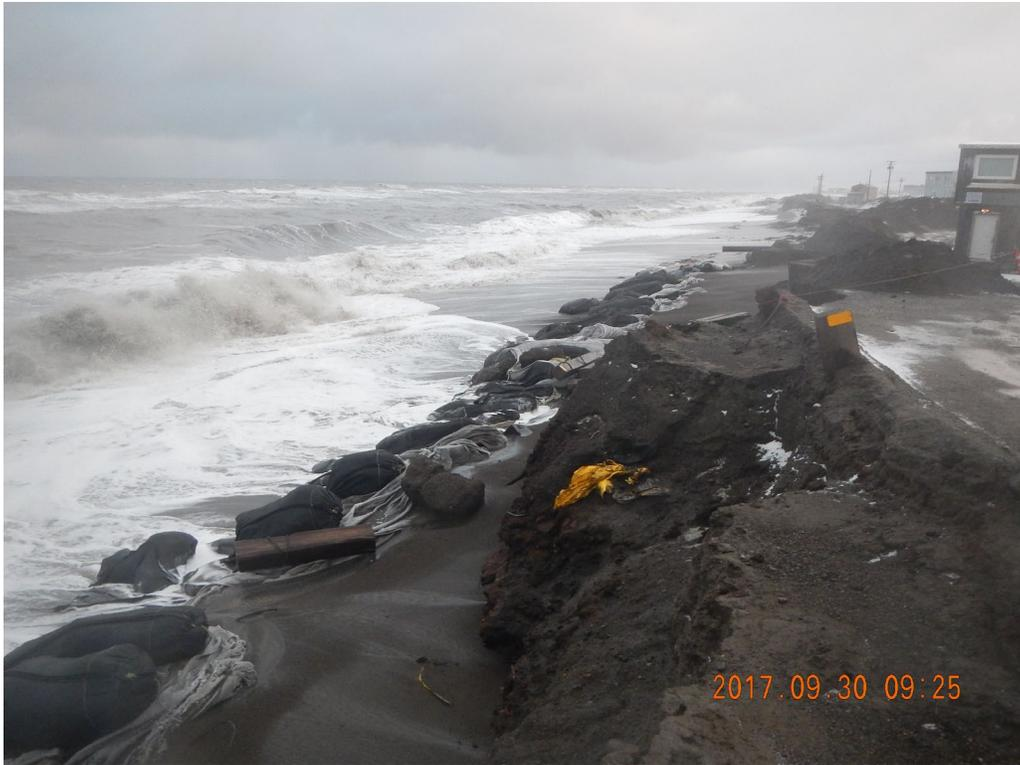
**Figure 16. Erosion along Bluff Threatening Egasak Street in Barrow (Sept 2017)**
