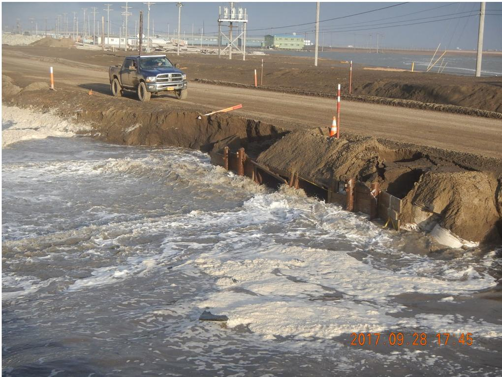
**Figure 15. Flooding of Middle Salt Lagoon Outfall and Erosion along Stevenson Street (Sept 2017)**
