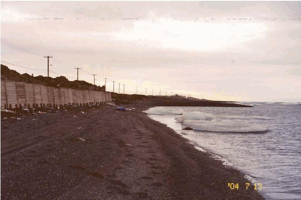
**Figure 23. Wooden Utilidors Backfilled with Local Material**
