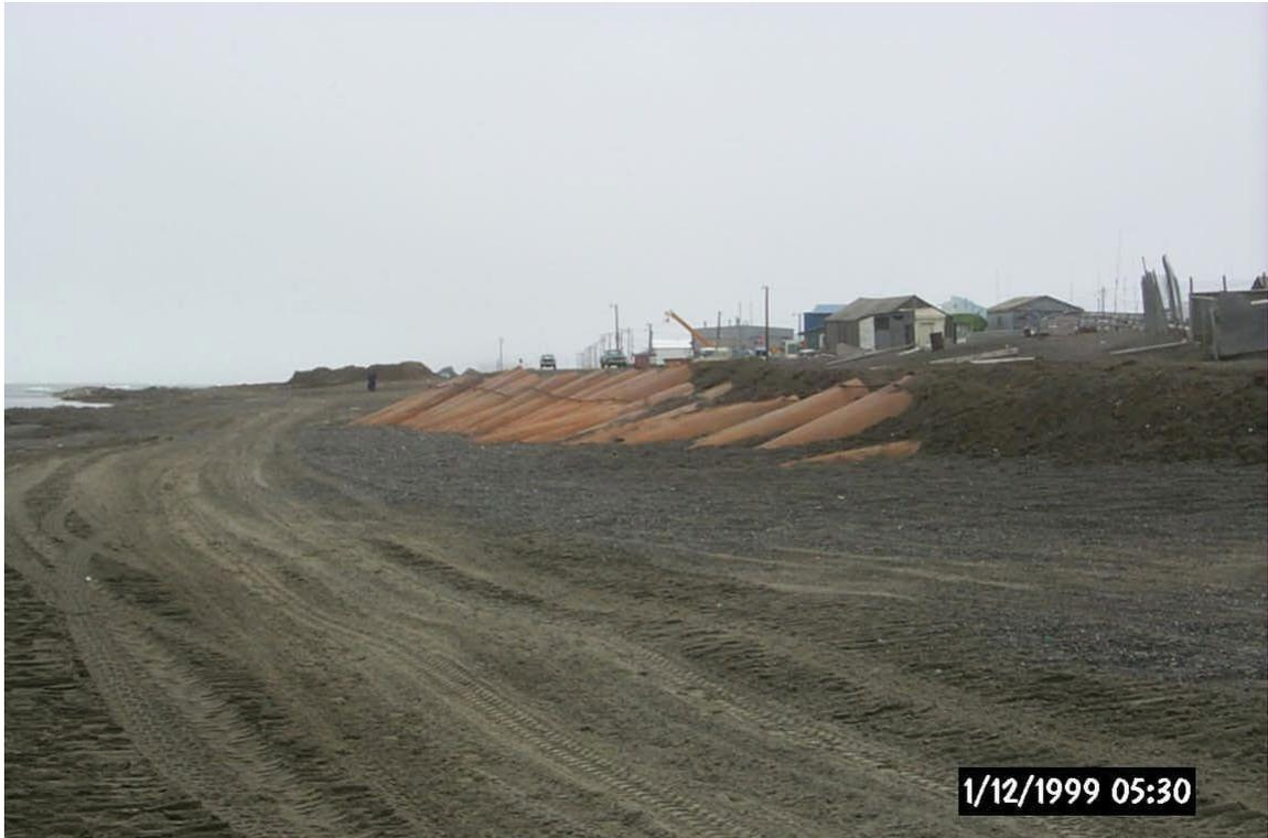
**Figure 24. Tar Barrels Laid on Beach at an Angle**
