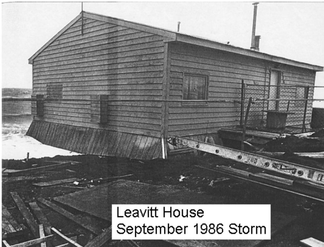
**Figure 8. Undermining of Structure from Erosion**
