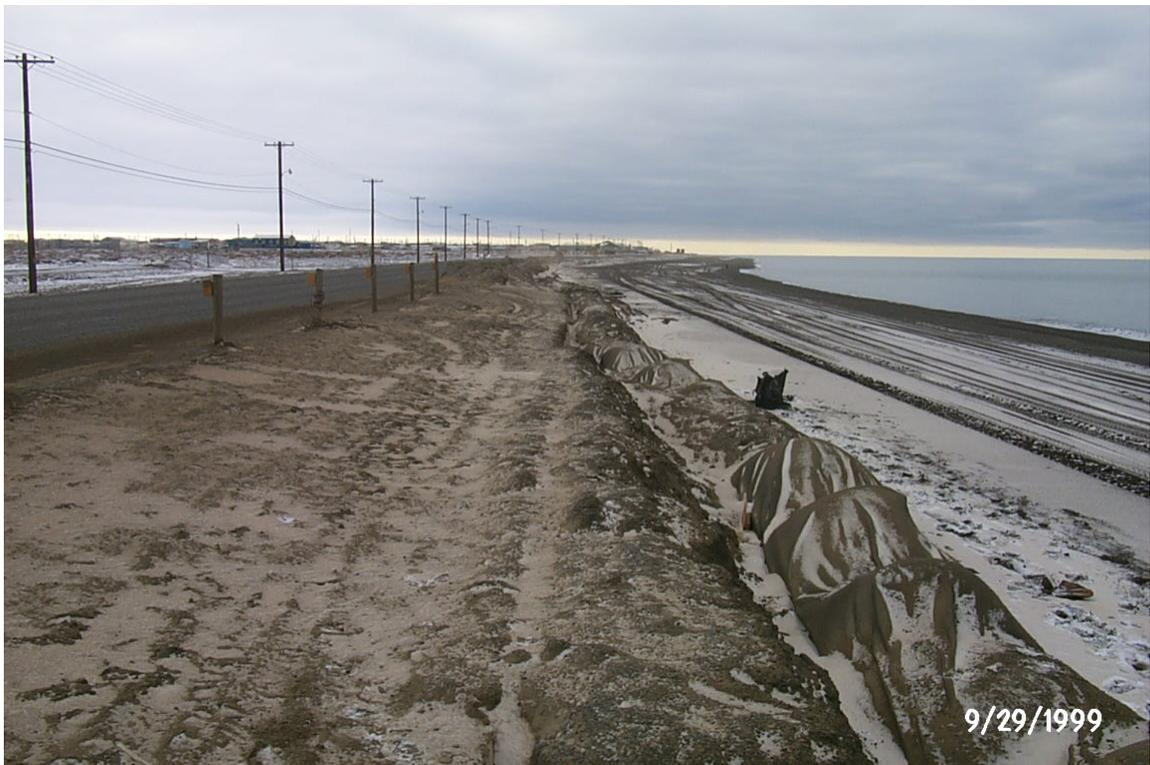
**Figure 25. Geotextile Tube Risk Reduction**
