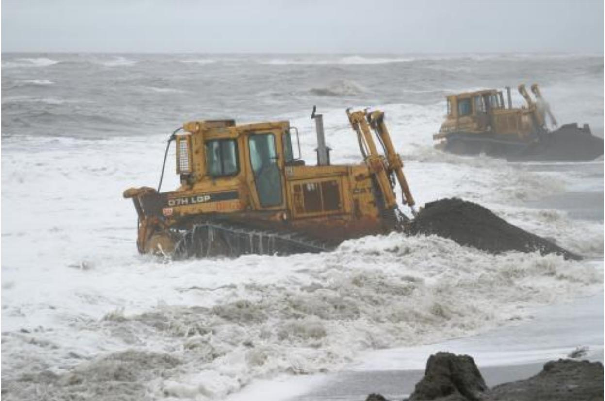
**Figure 19. Bulldozer Pushing Beach Material During Heavy Surf**
