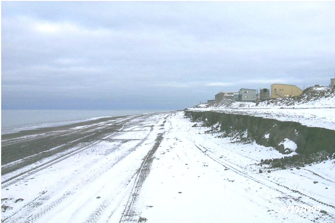
**Figure 21. Remains of Beach Nourishment after Storm. The dredge Program was never Completed. The North Slope Borough's Dredge Grounded During a Storm in 2000.**
