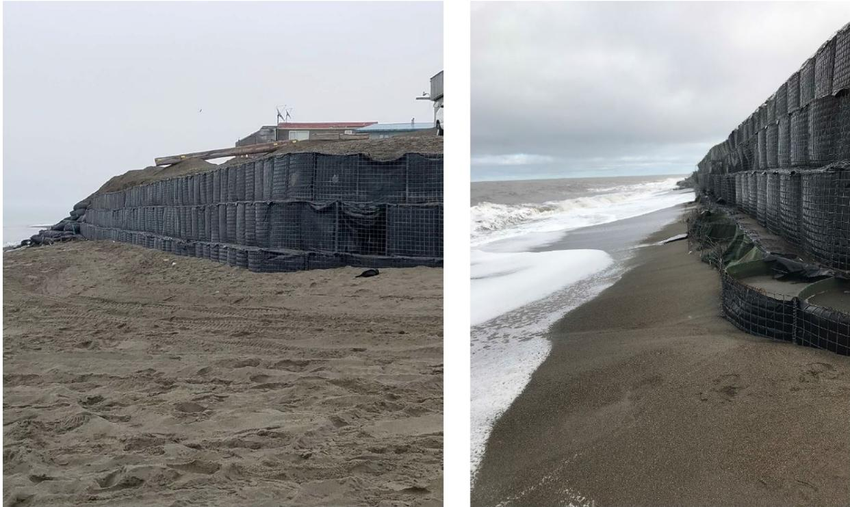
**Figure 26. HESCO Baskets in front of Barrow near The Fur Shop from September 2017 (Left) and after the August 2018 Event (Right)**
