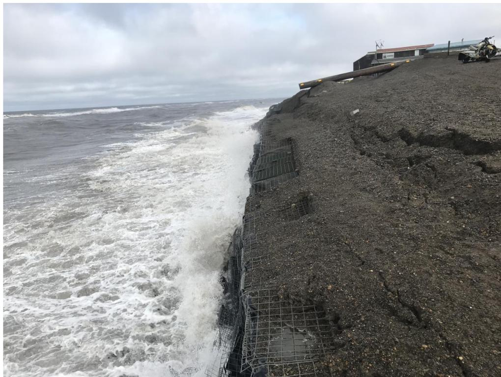
**Figure 17. High Total Water and Run-up that Failed the Gabion Baskets along the Bluff in Barrow (Aug 2018)**
