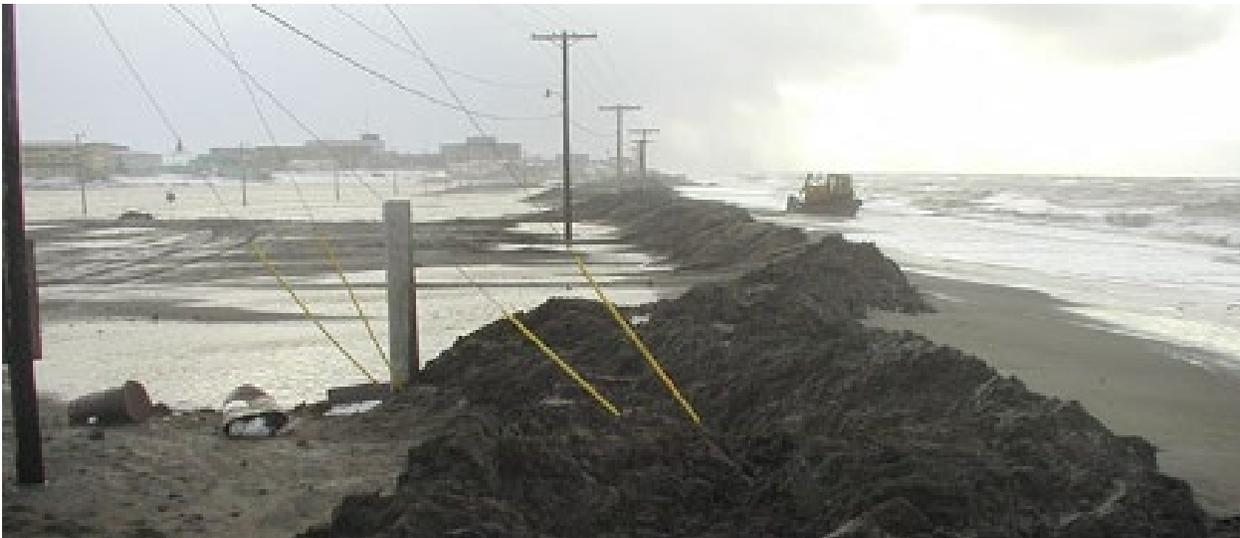
**Figure 18. Bulldozer Working on the Beach Building Berms**
