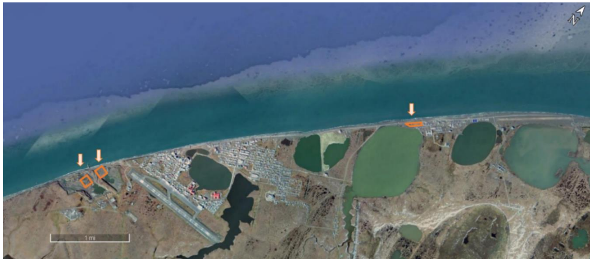
Figure 3. Staging Area and Barge Offloading Areas
