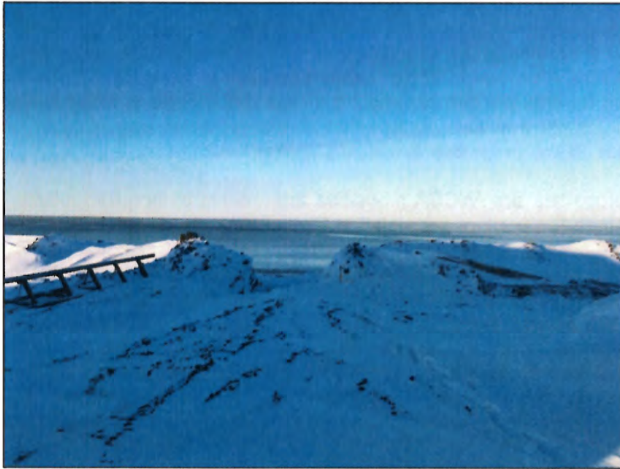
Figure 28. Break in the sacrificial berm for public beach access in Barrow, Alaska.
