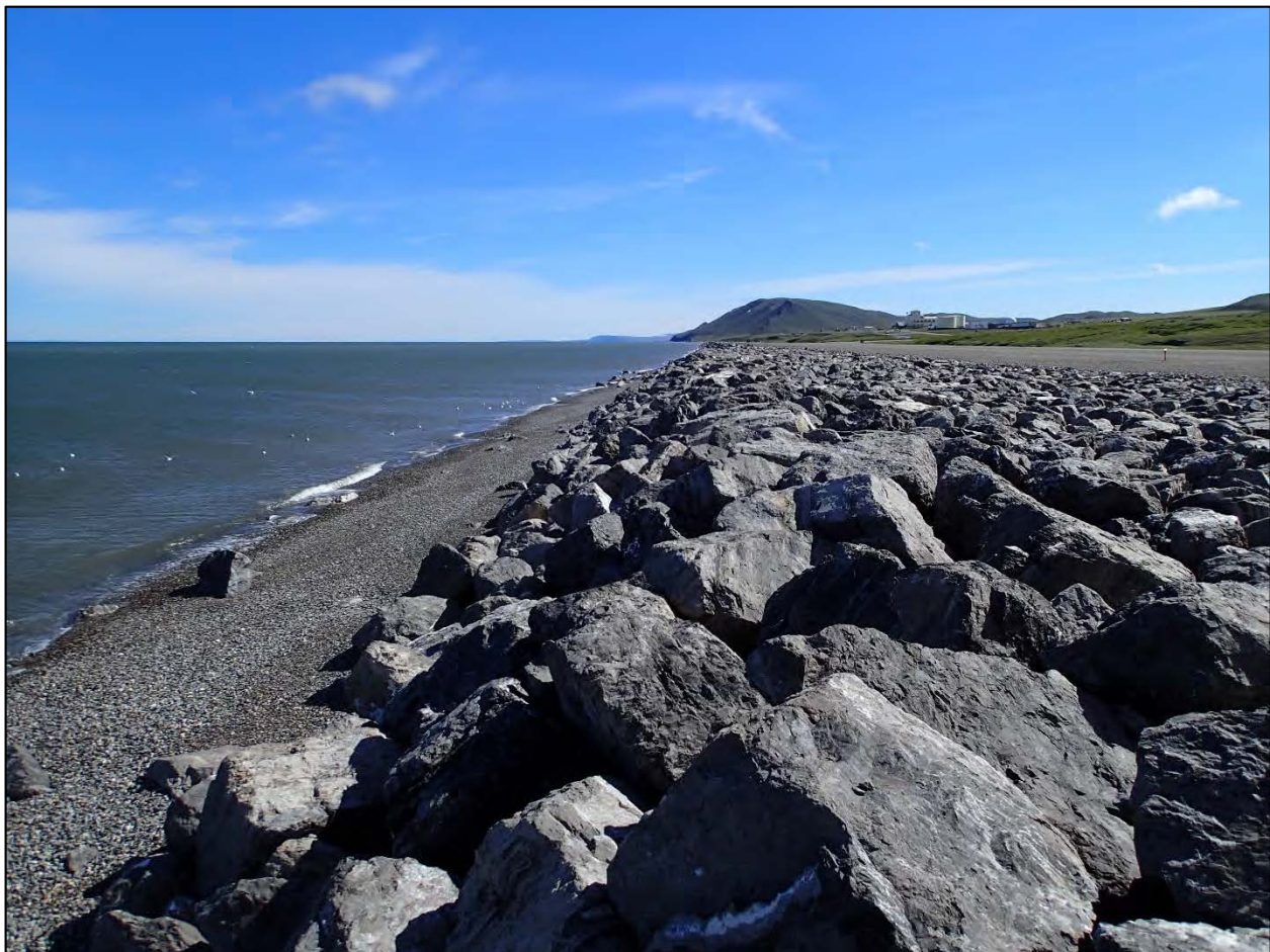
Figure 8. An example of a rock revetment from a Corps project on Cape Lisburne. Armor rocks shown are approximately 3.5 tons each. Note that there is no high natural bluff which is present in Barrow.
