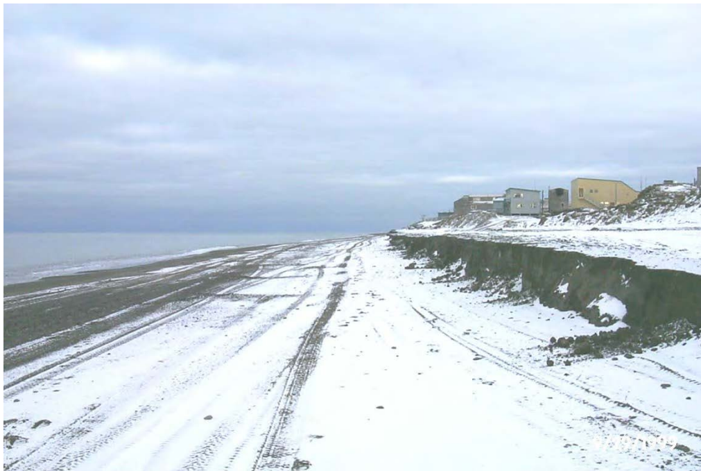
Figure 17. Remains of Beach Nourishment After Storm. The Dredge Program Was Never Completed. The North Slope Borough's Dredge Grounded During a Storm In 2000.
