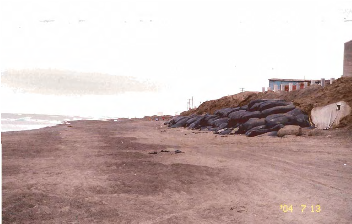
Figure 18. Supersack Revetment.
