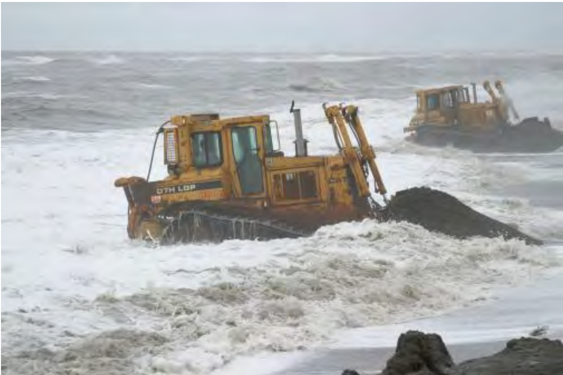
Figure 15. Bulldozer Pushing Beach Material During Heavy Surf.
