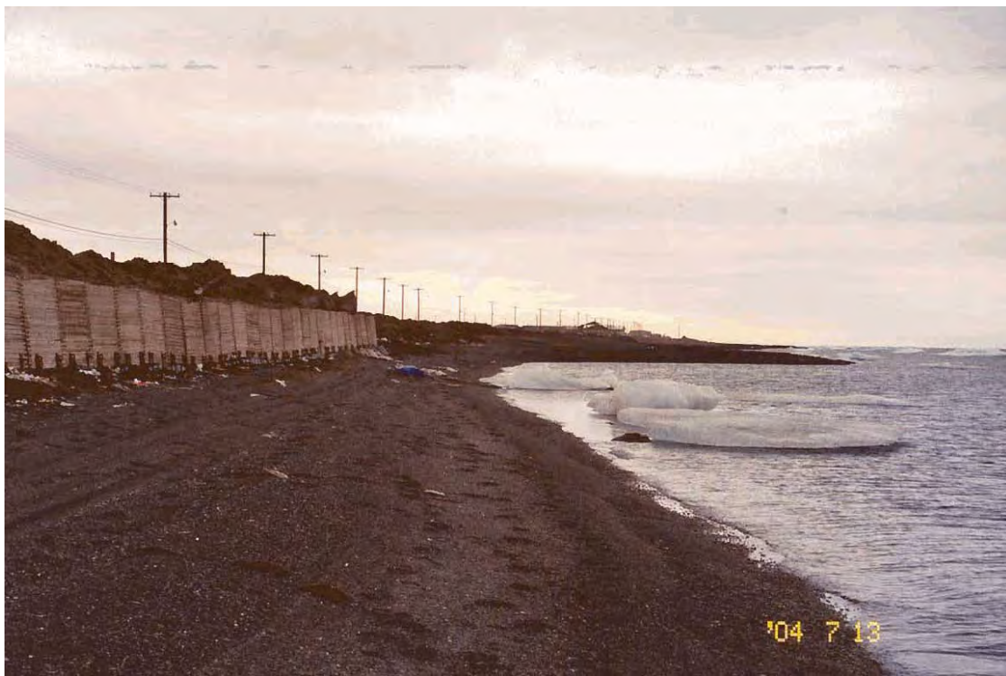
Figure 19. Wooden Utilidors Backfilled with Local Material.
