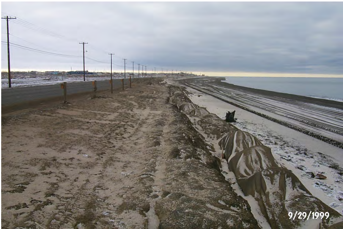
Figure 21. Geotextile Tube Protection.
