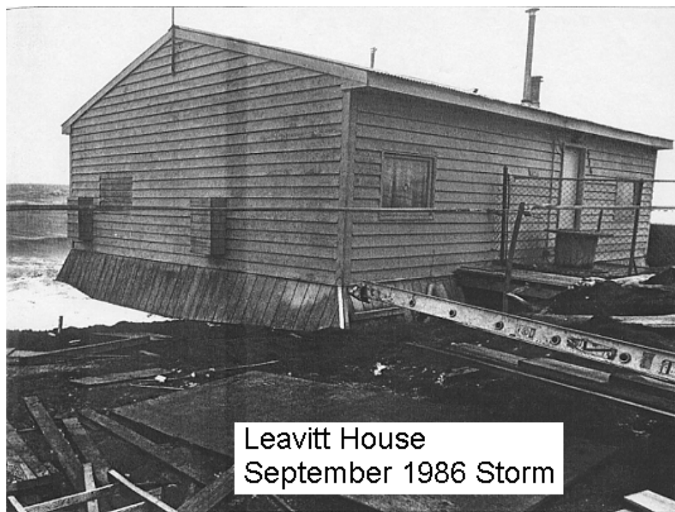
Figure 8. Undermining of Structure From Erosion.
