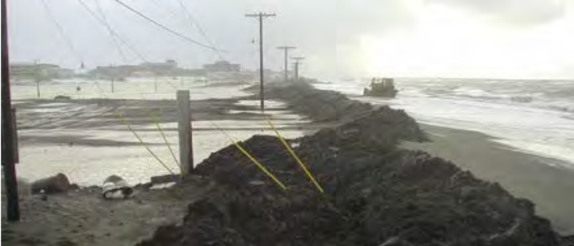
Figure 14. Bulldozer Working on the Beach Building Berms.
