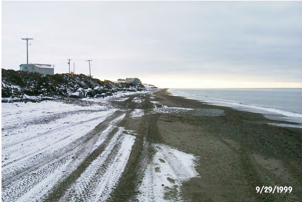
Figure 16. Sacrificial Berms Placed Along Road.
