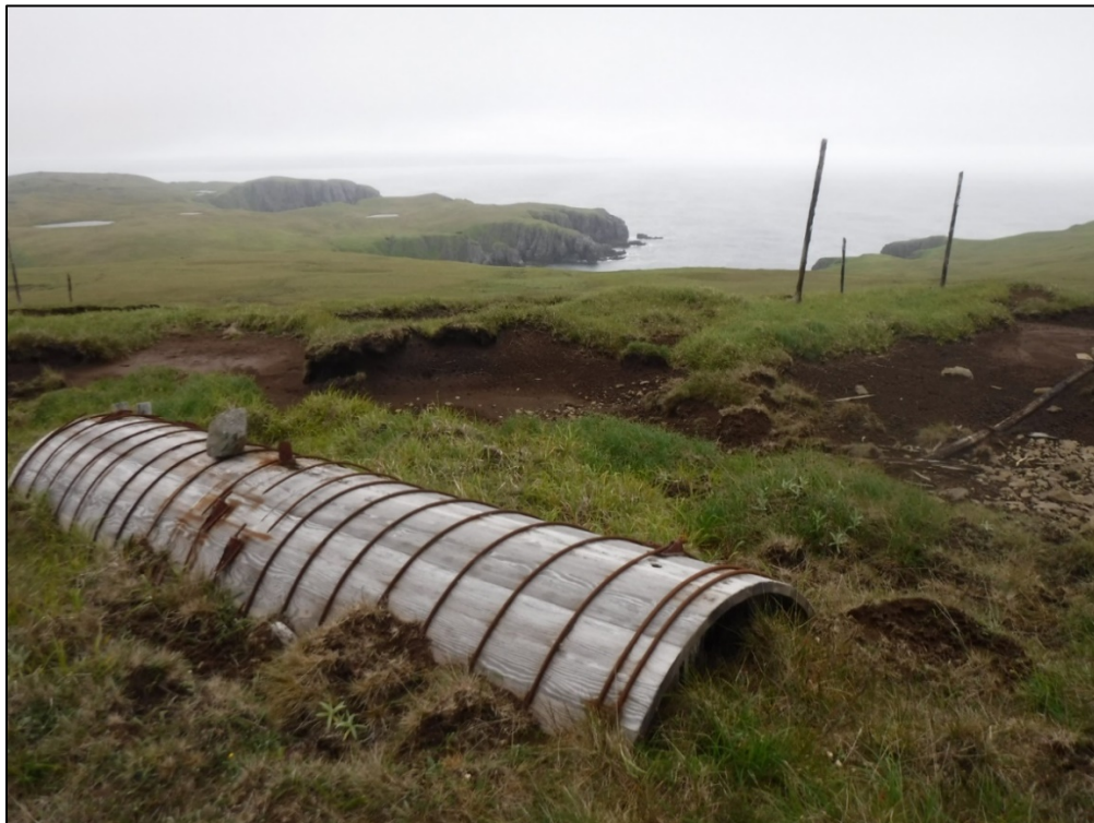
Figure 4. A partially sunken AST, located on the previous map as AST 2. The picture includes the extensive erosion which is present throughout the site.
