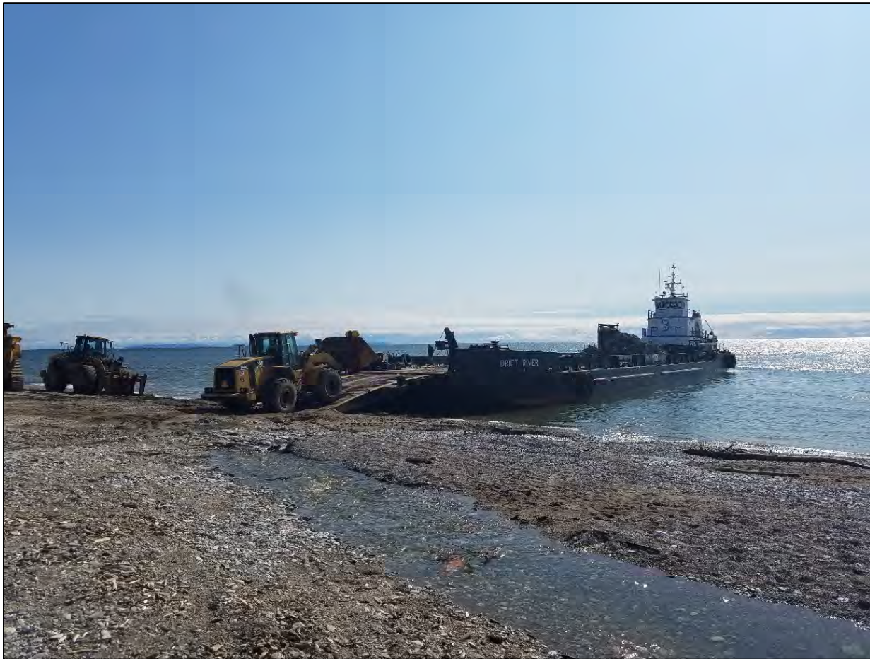
Figure 34. Offloading of a Materials Barge on Elim Beach (August 2018).
