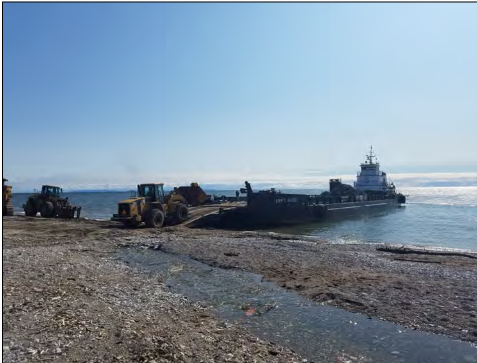
Figure 46. Offloading of a materials barge on Elim Beach (August 2018)
