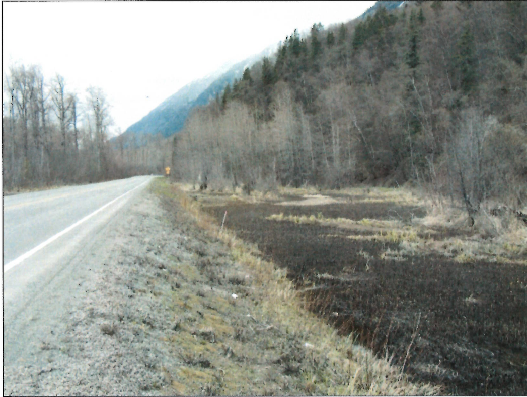
Figure 3. Overview of PMP 17.7 on east side of highway, pipeline was located along the right edge of the wetland, view NW (M. Grover 2007).
