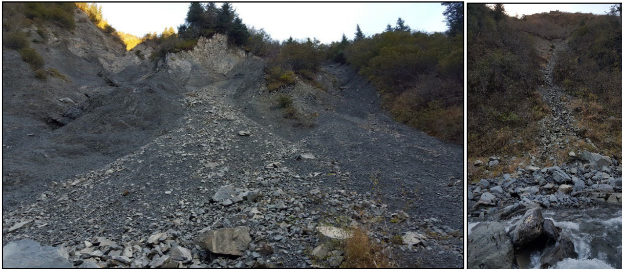
Figure 9. Lowell Canyon Weathered Rock Face and Slope Failures Upstream from Diversion Facility.
