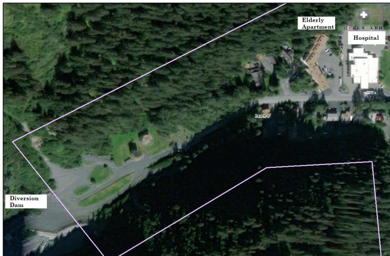
Figure 3. Seward Critical Infrastructure
