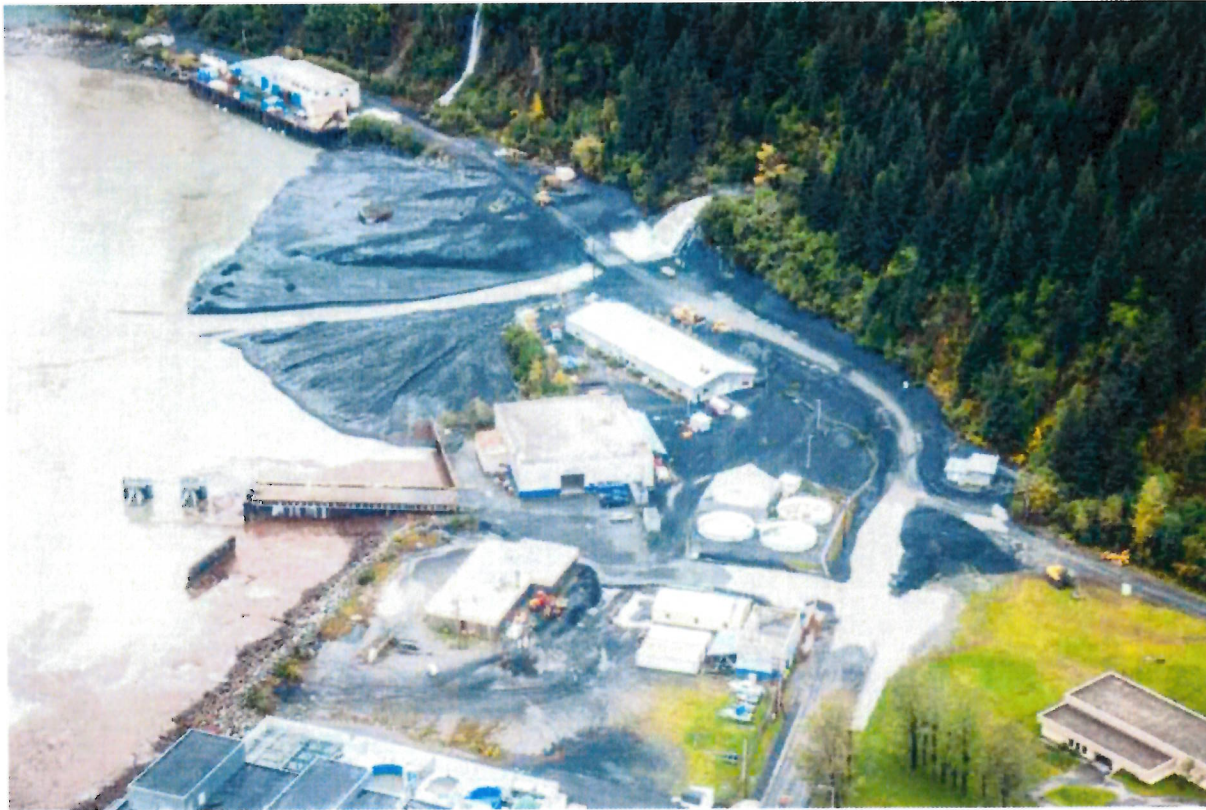
Figure 2. Existing Lowell Creek outfall terminus
