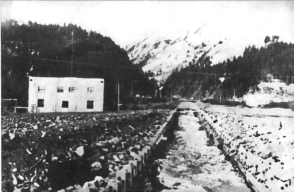
Figure 2. The Lowell Creek funnel structure built through Seward by the railroad (AHR Record #16122578).
