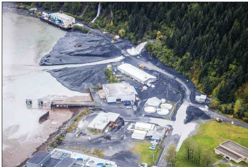
Figure 12. Tunnel Outlet Area during 2012 Flood.
