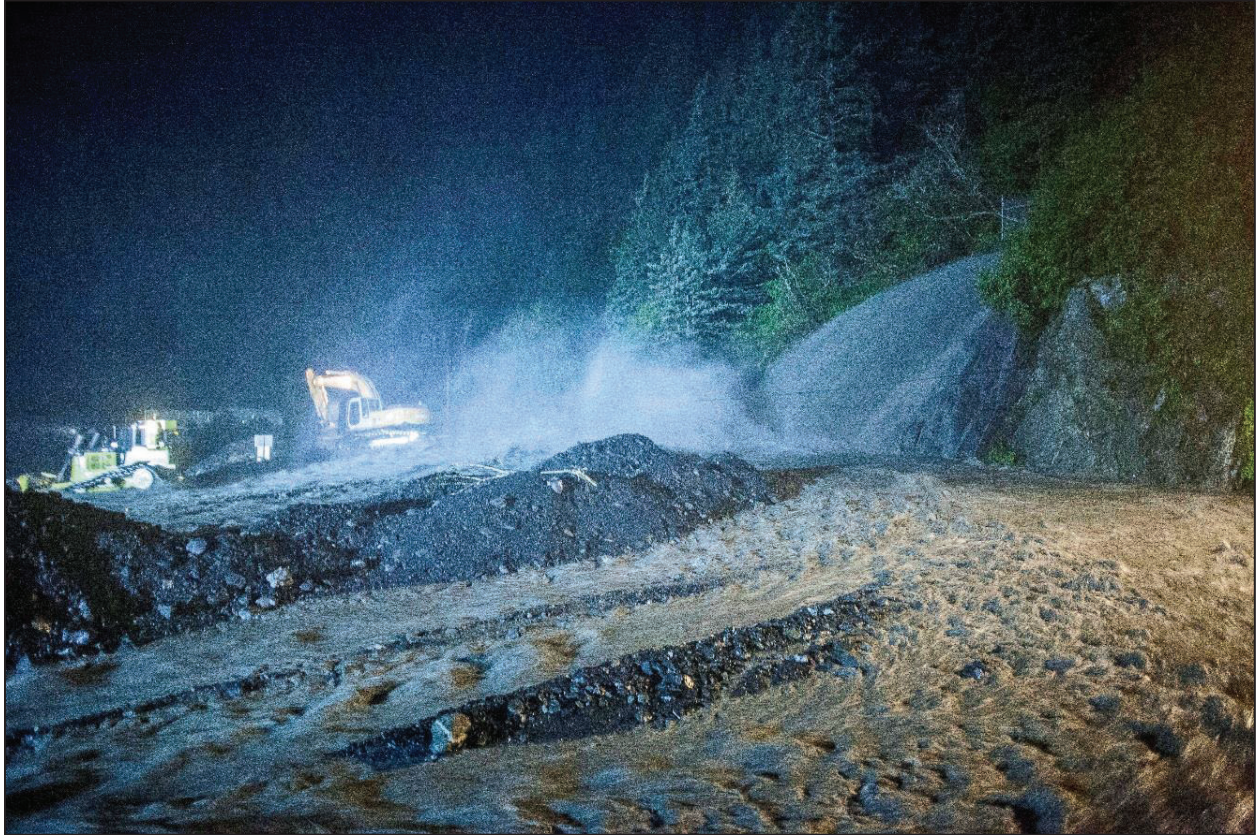
Figure 10. Heavy Equipment Removing Sediment from Tunnel Outfall During 2012 Flood .
