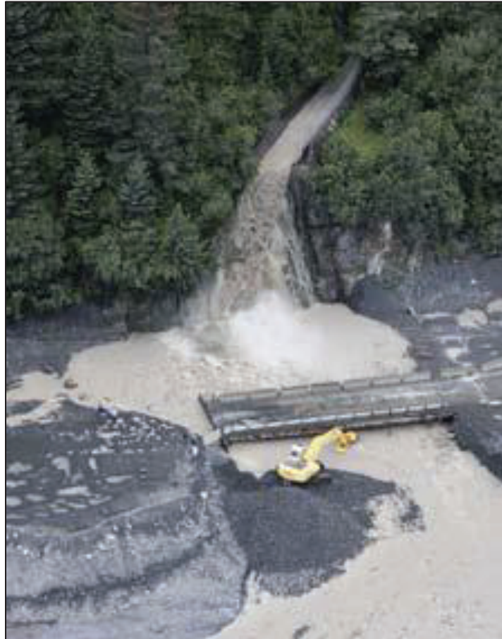
Figure 11. Lowell Creek Bridge during 2009 Flood.
