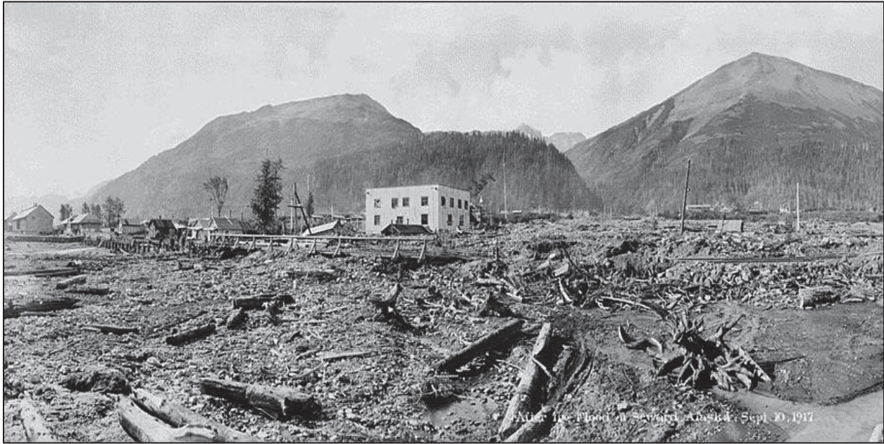
Figure 5. Flood of 1917 with Building Buried to Second Story in Debris.
