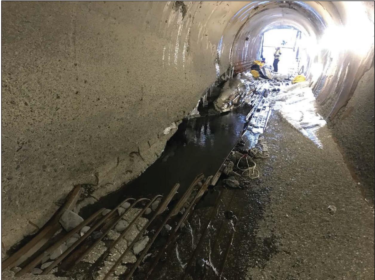
Figure 9. Large Scour Hole in Floor of Tunnel Repaired During 2017 Repairs.
