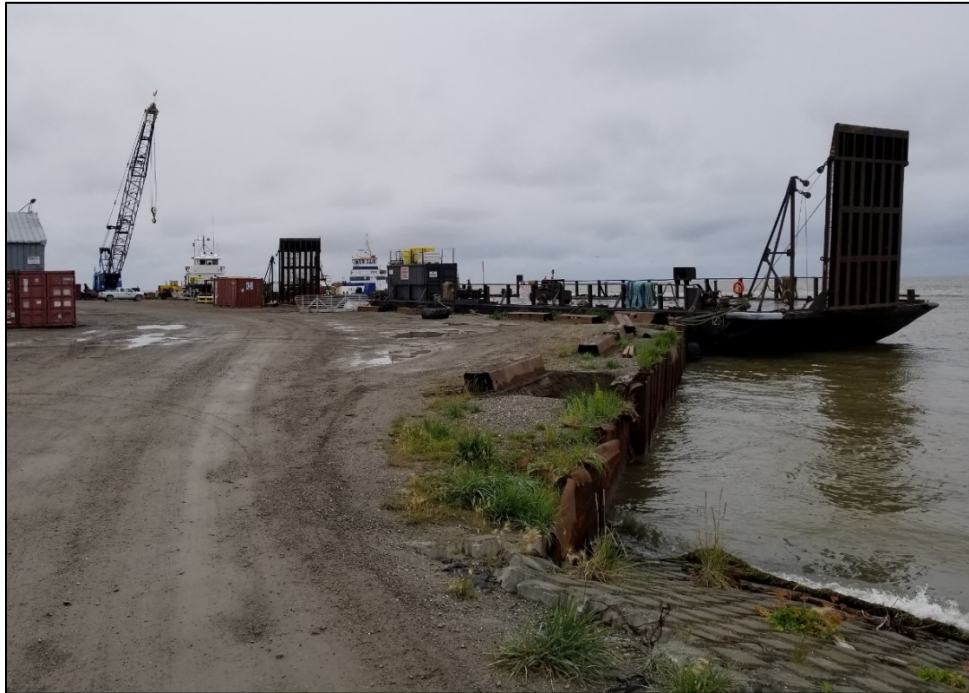
Figure 12. Tug and Barge docking alongside at Kotzebue
