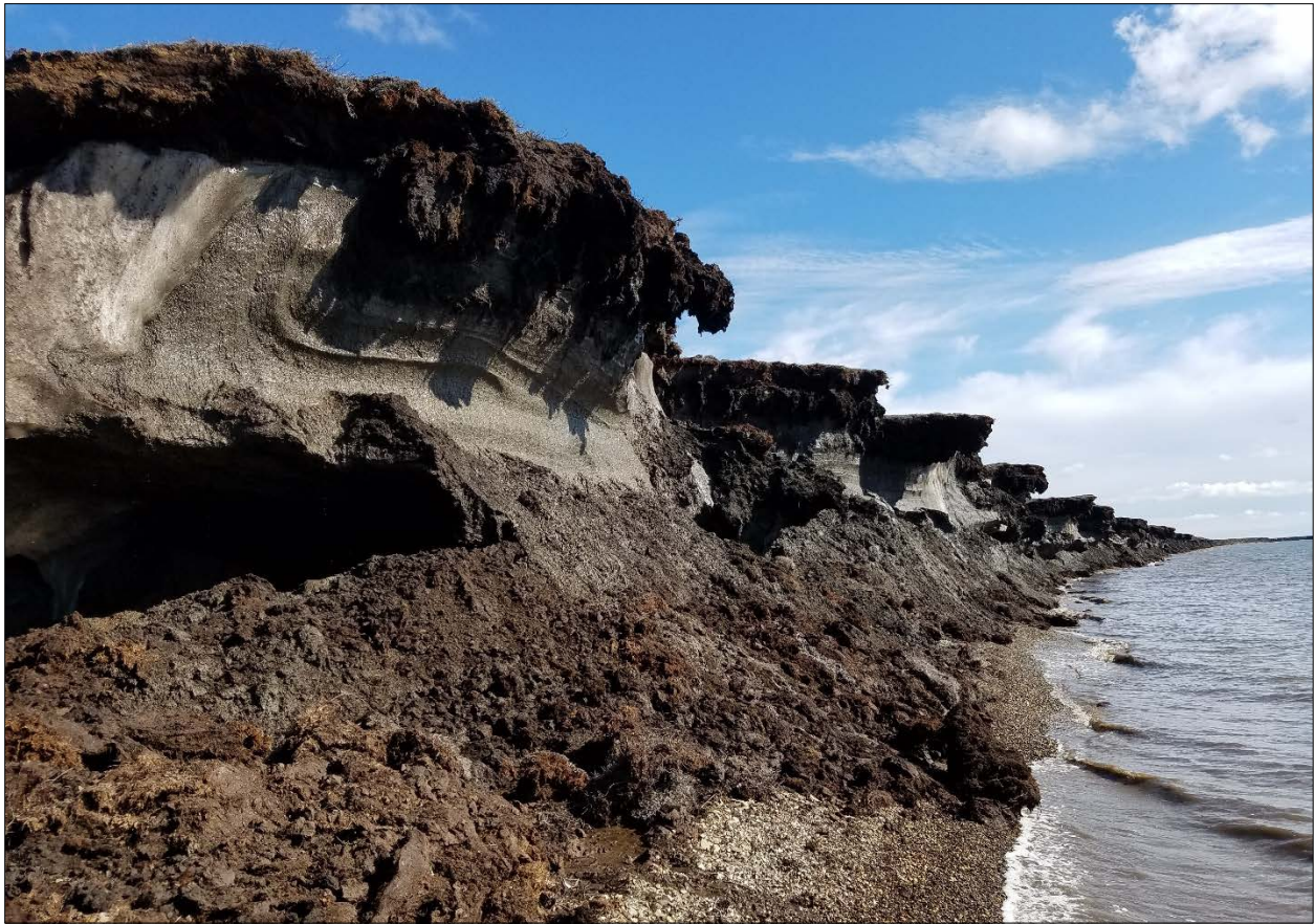
Figure 9. Beach bluff face in project area in 2016, showing ice lenses and active erosion.
