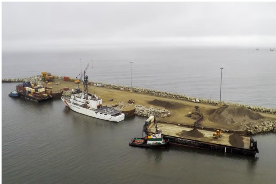
Figure 29 Gravel loading operation at the Westgold dock via conveyor
