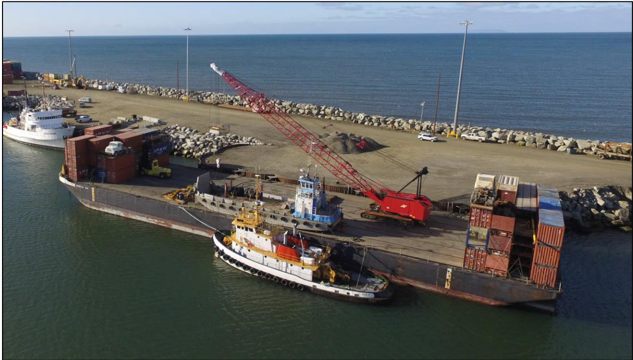
Figure 11. Typical Cargo Barge with organic crane at the Port of Nome Westgold Dock
