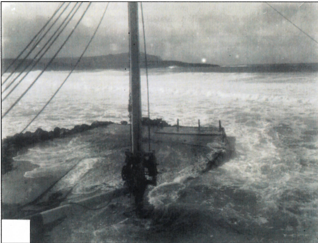
Figure 8: Historic photo of the small dock (XPI-195), date unknown, catalog number RG22-95-ADMC-2863 (NARA 2018).
