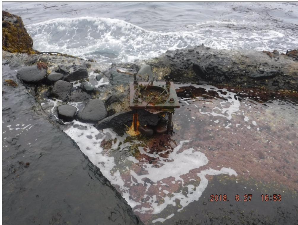
Figure 16. An exposed metal base for a wooden lever joist is located just off the St. George Outside Landing (XPI-194) near where the dock connects to the shoreline (Sparaga 2018).
