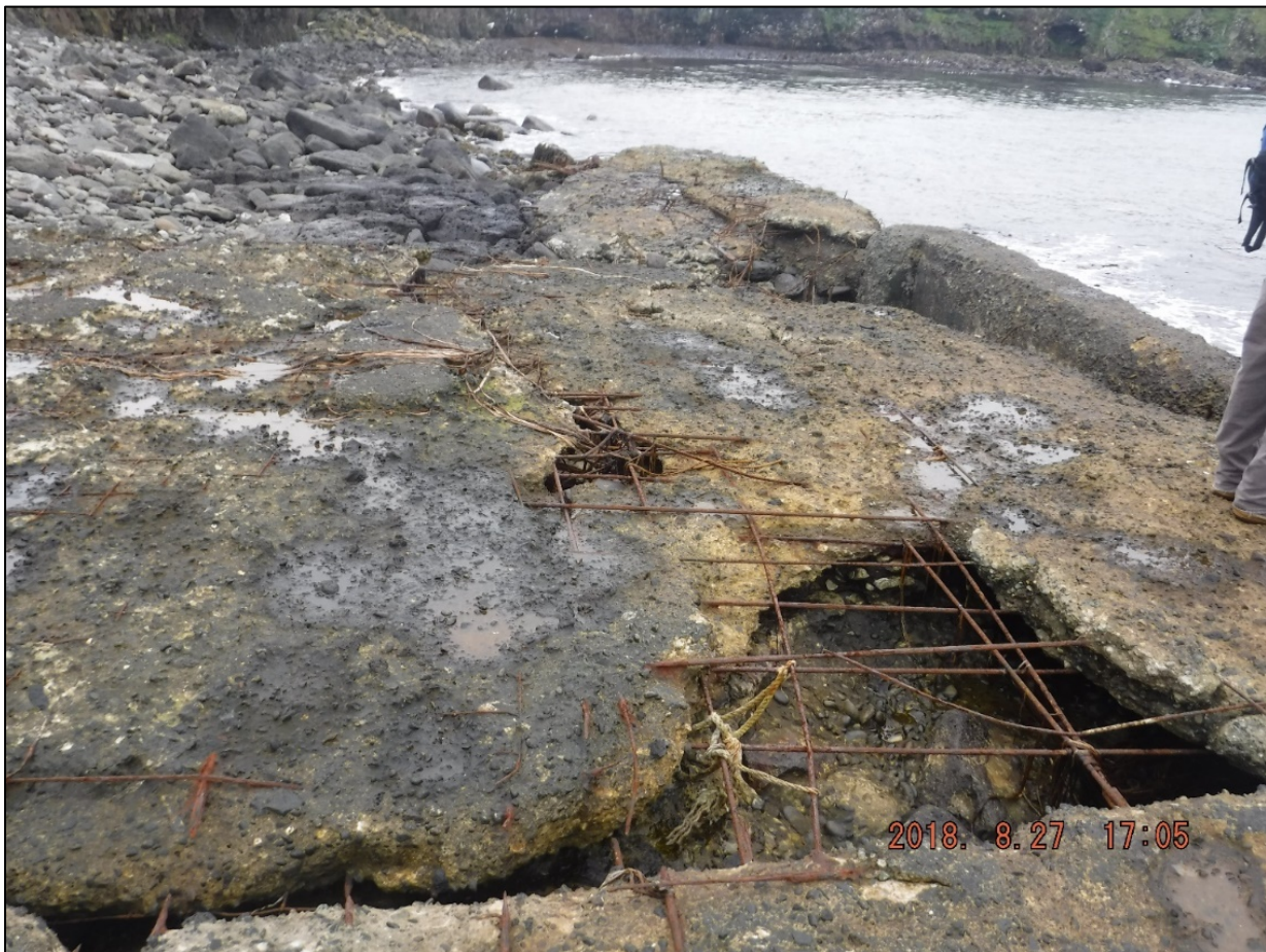
Figure 11. The weathered reinforced concrete on the St. George Inside Landing (XPI-195). Interior sections of the dock are exposed and show substantial concrete degradation and loss of fill.
