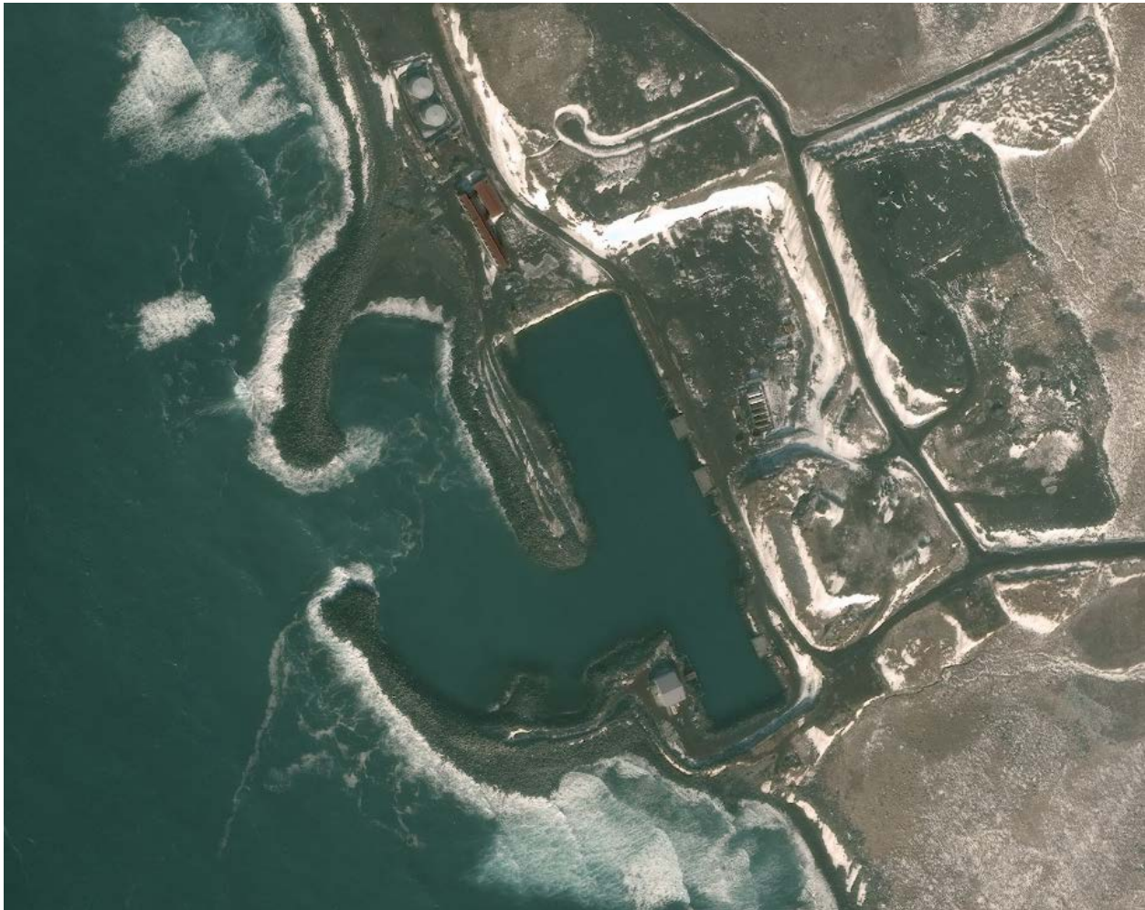
Figure A-3: St. George Harbor aerial image.
