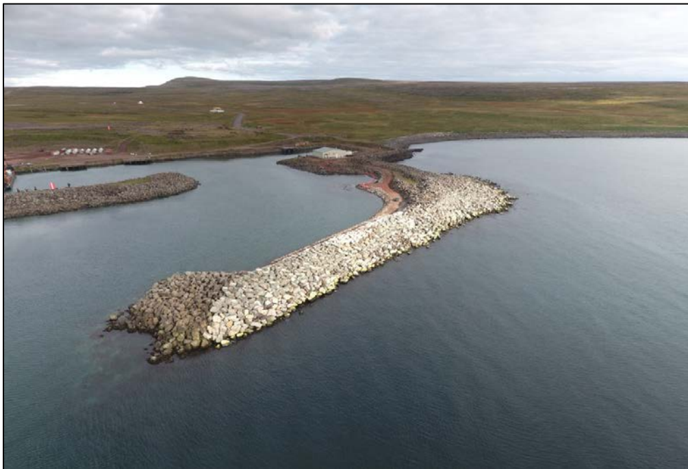
Figure C-6: Breakwater After Repairs, 2017
