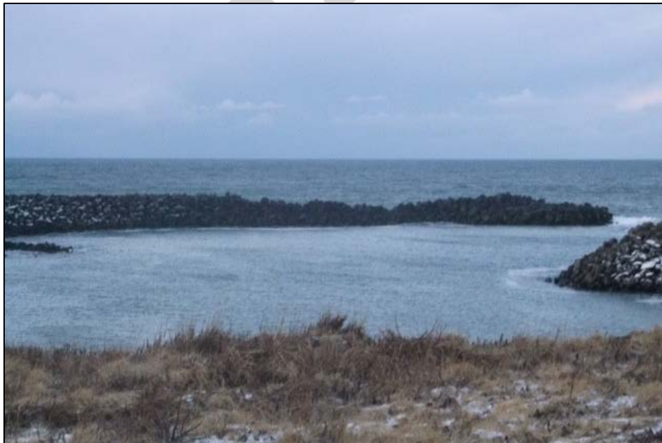
Figure C-5: Breakwater After December 2015 Storms
