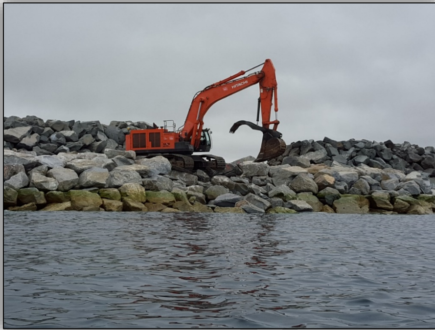
Figure C-9: Locking Armor Stone into the Breakwater
