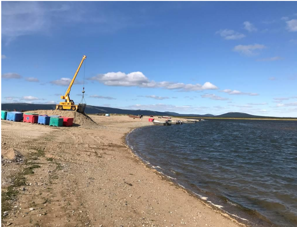
Figure 8. NSEDC Fish Buying Station and Safe Moorage up Kwiniuk River at Moses Point (August 2018)
