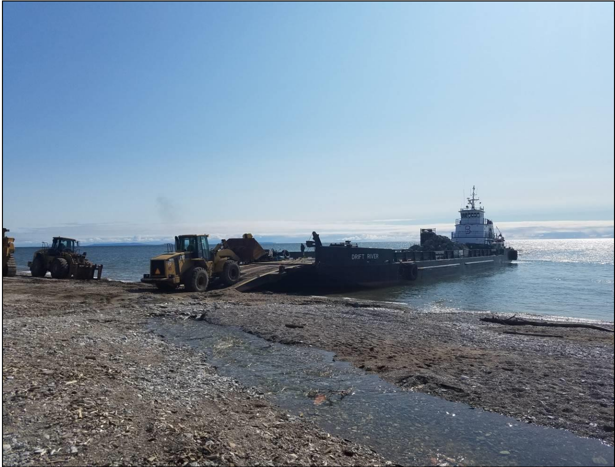
Figure 49. Offloading of a Materials Barge on Elim Beach (August 2018)
