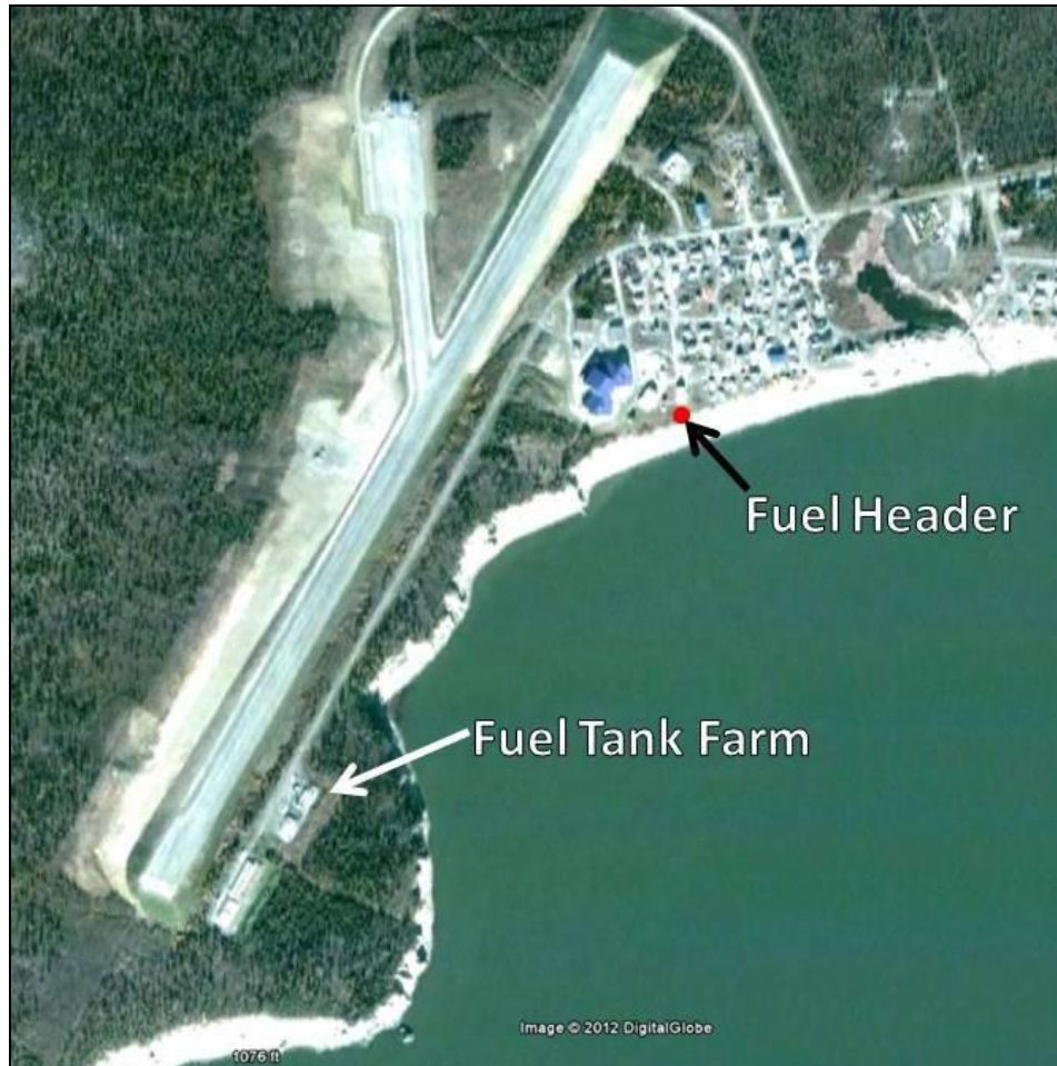
Figure 20. Fuel Tank Farm Relative to Fuel Header
