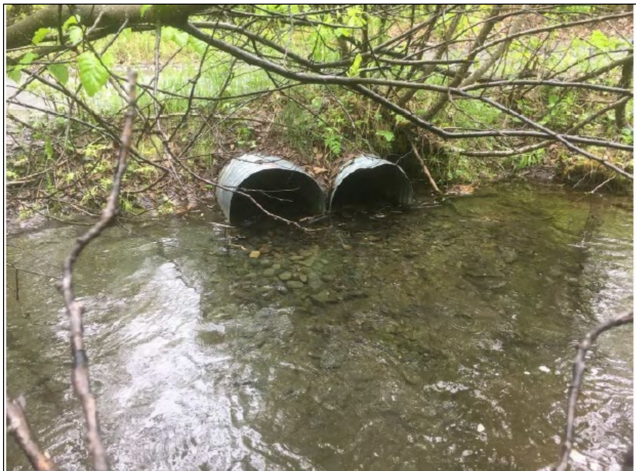
Figure 23. Old Corbin Creek culverts under the ALPETCO trail.
