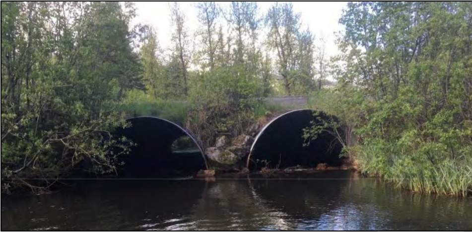
Figure 14. 12.75 ft. diameter culverts on Robe River under the Richardson Highway.
