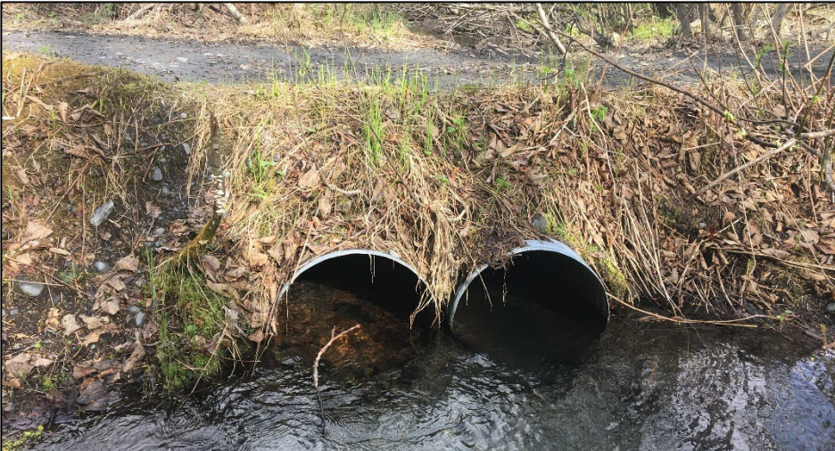
Figure 15. 24-inch diameter culverts on Old Corbin Creek under the ALPETCO trails.
