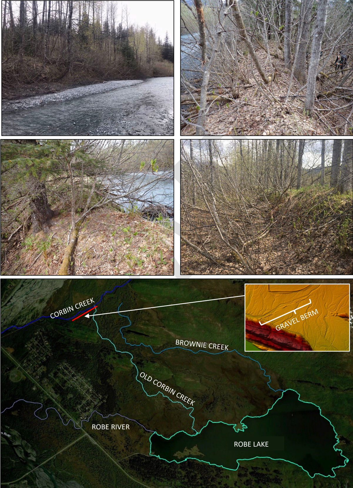
Figure 11. Photographs and LiDAR imagery of gravel berm along Corbin Creek.
