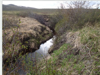
Drainage Channel with steep sides, heavy vegetation
