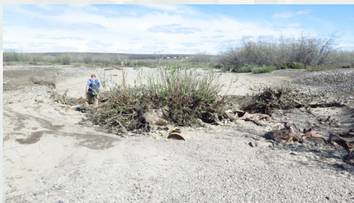
Exposed Debris during June 2019 Landfill Inspection
