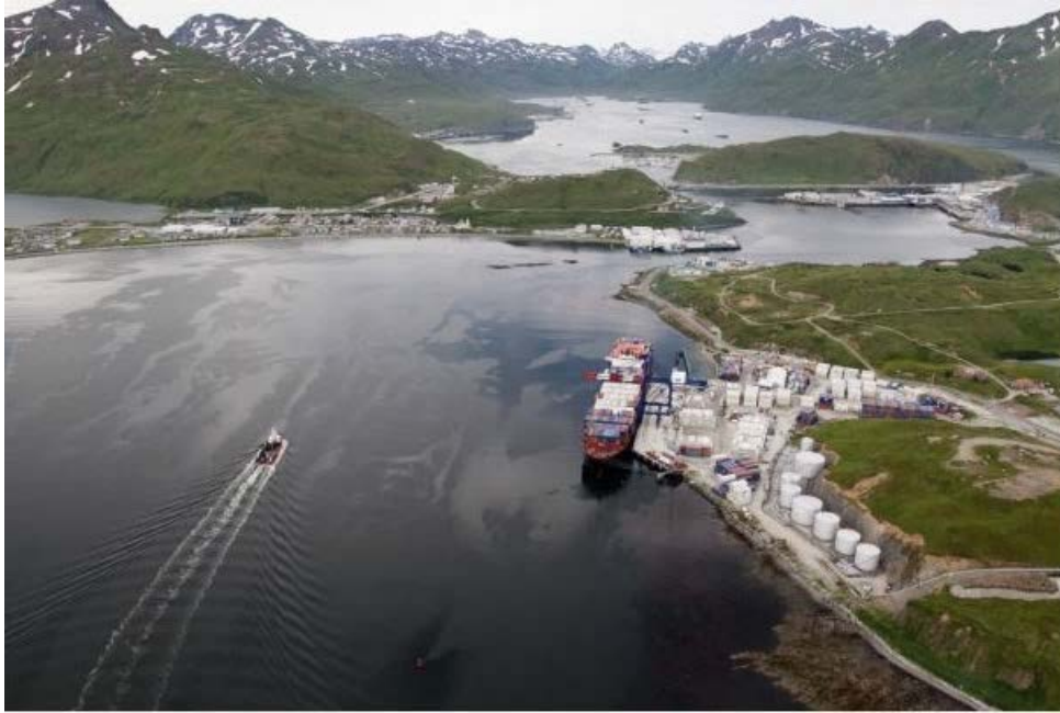
Figure 10 APL Dock looking south
