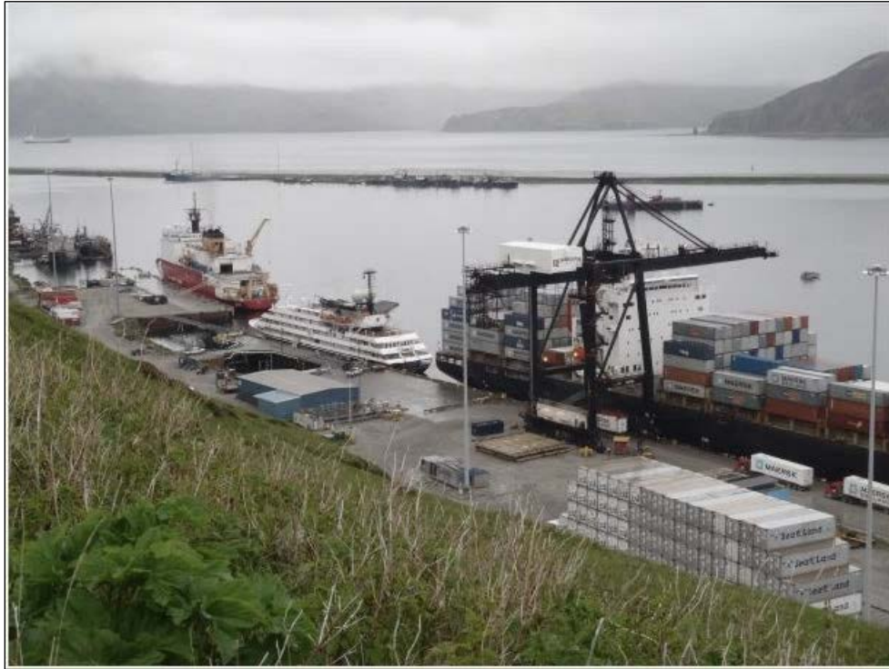
Figure 21. Unalaska Marine Center (UMC) and USCG Dock
