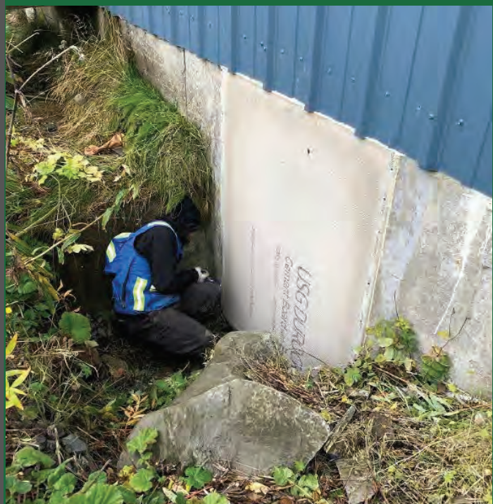
Photo 5. 2019 Building 551 Crawl Space Covers
