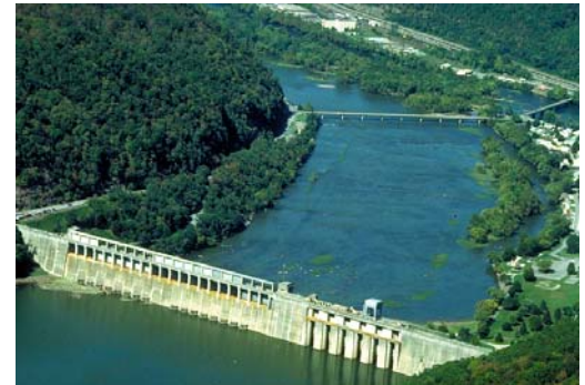
Bluestone Lock and Dam, WV
