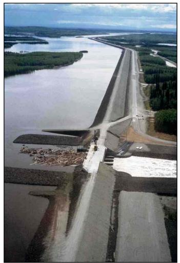
Since Moose Creek Dam began operations in 1981, the Corps has successfully managed 20 flood events. The largest impoundment occurred in 1992 when the flow in the Chena River was reduced for 18 days.
