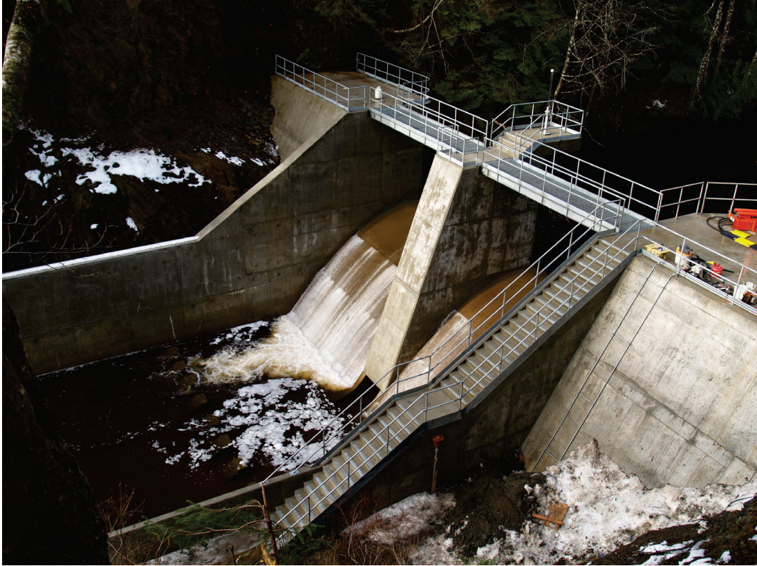
Downstream of Kake Dam during construction, January 2007
