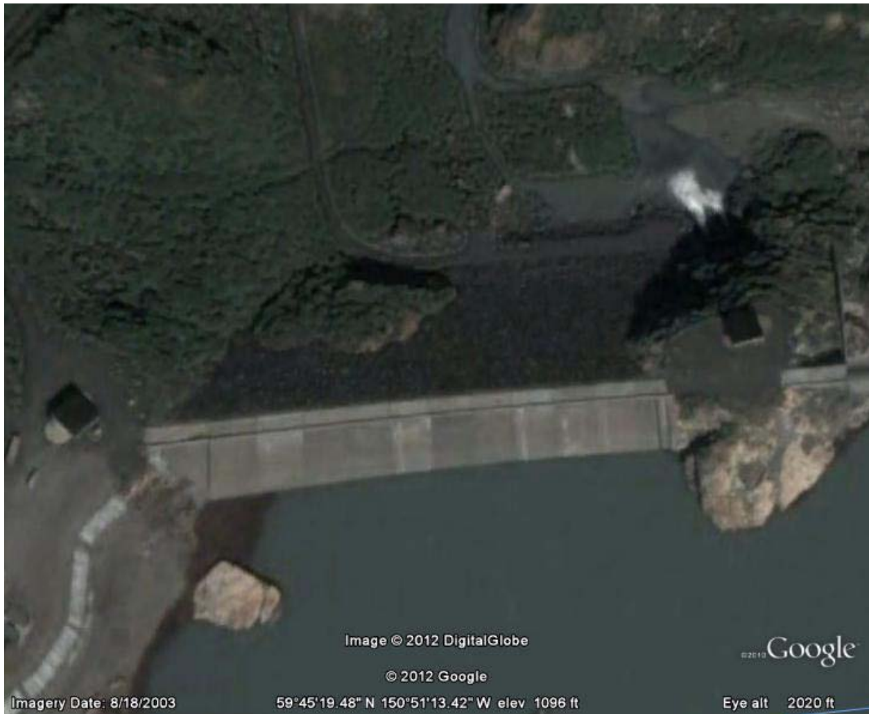
Bradley Lake Dam overhead Google image, 18 August 2003.
