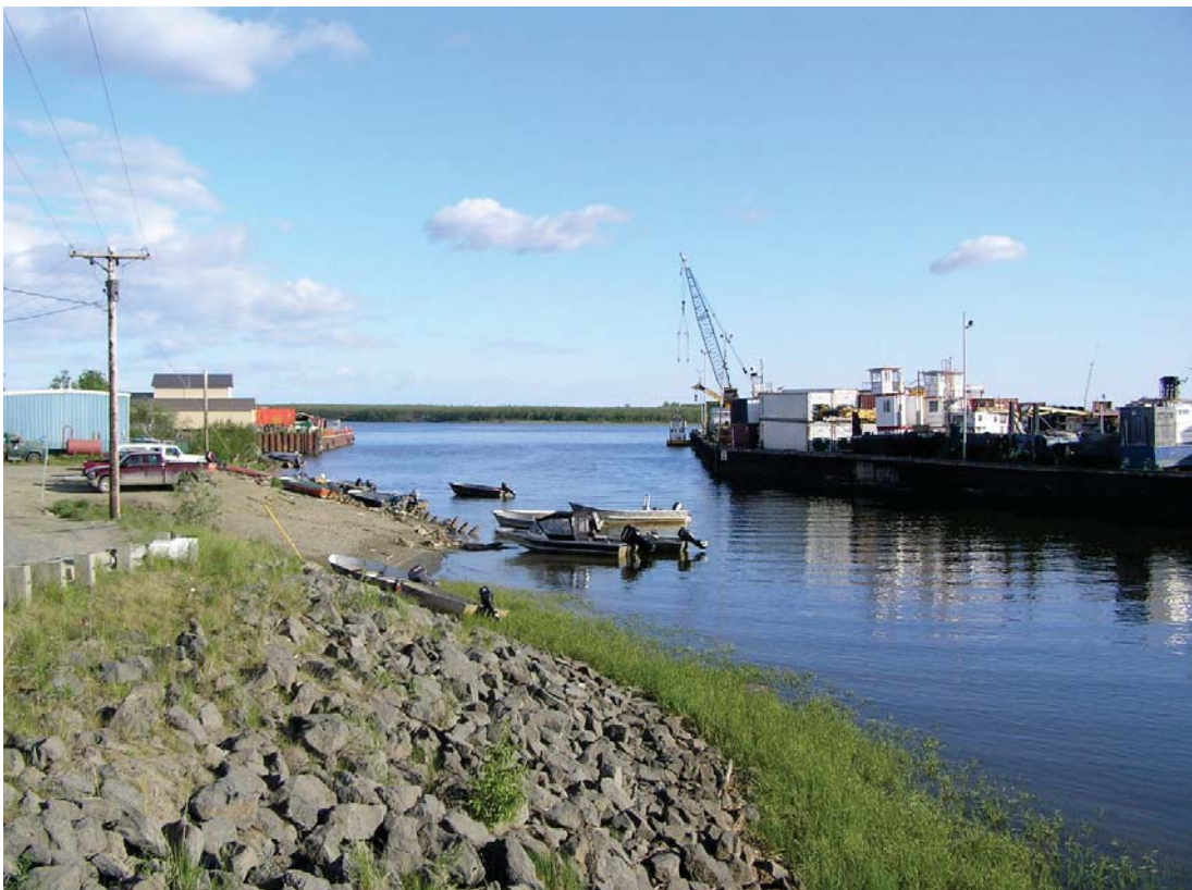
Bethel Bank Stabilization along Brown's Slough, June 2007
