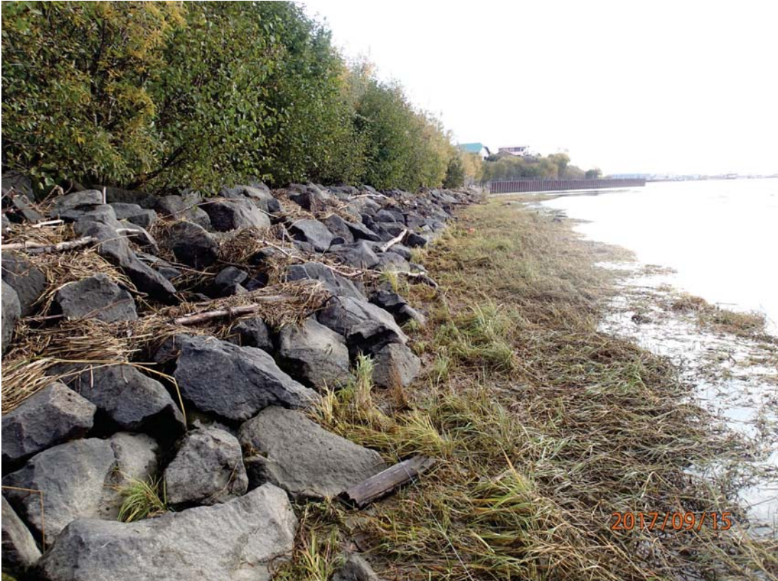
Typical rock revetment and seawall at downstream end of Mission Road, 2017
