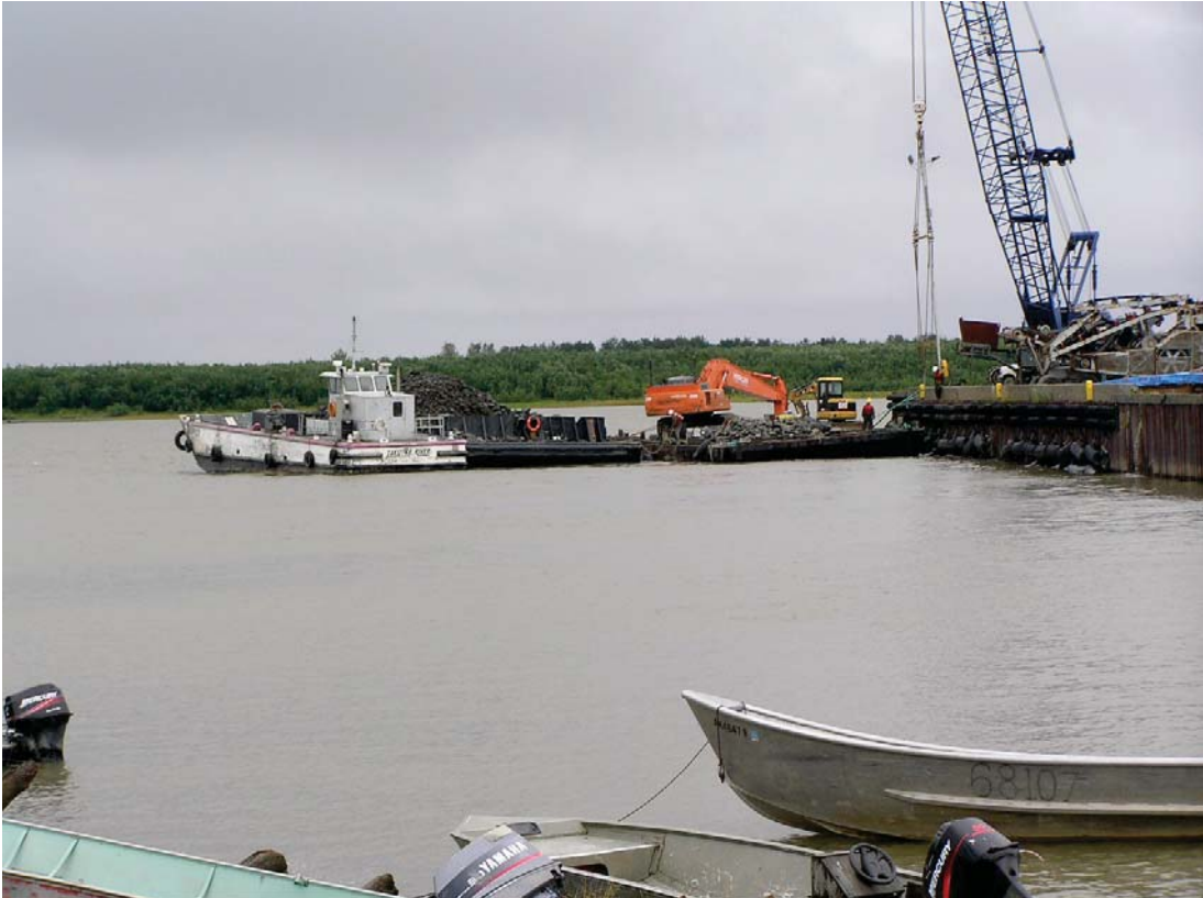
Placement of riprap, August 2007
