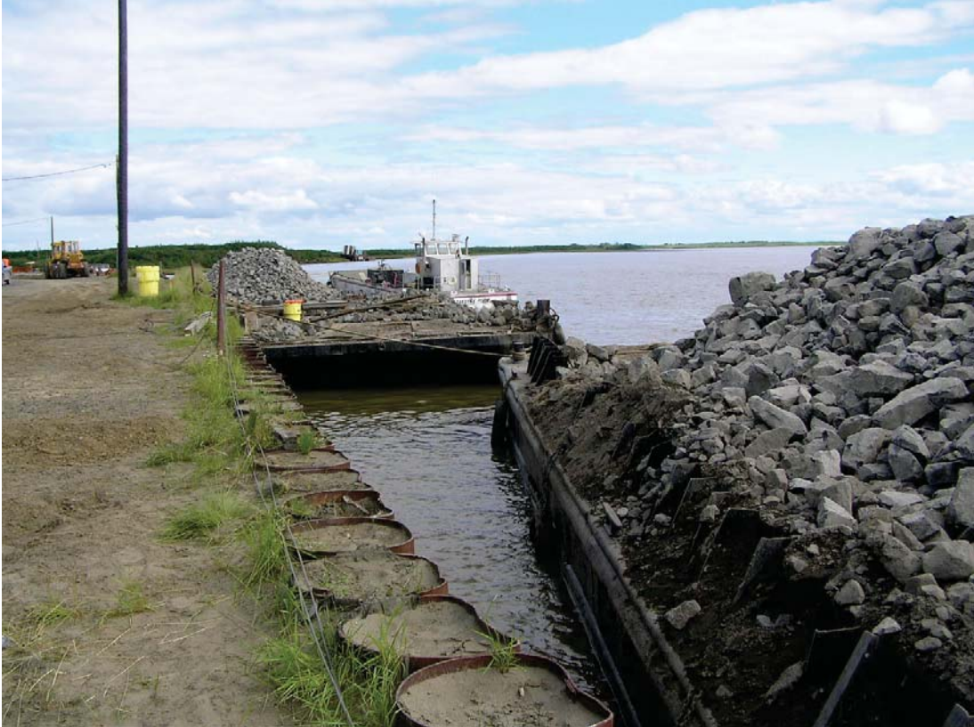
Riprap transport for the Bethel Bank Stabilization project, July 2007
