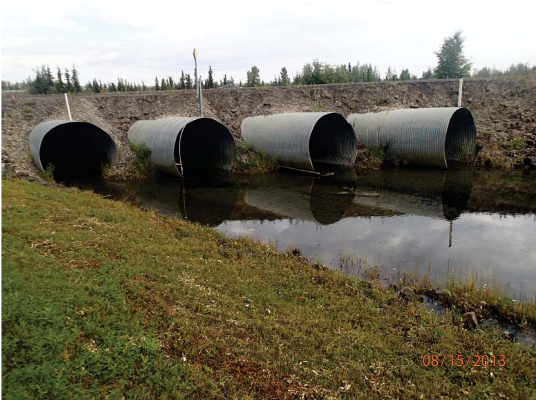
Culverts within the Tanana River Levee, August 2013
