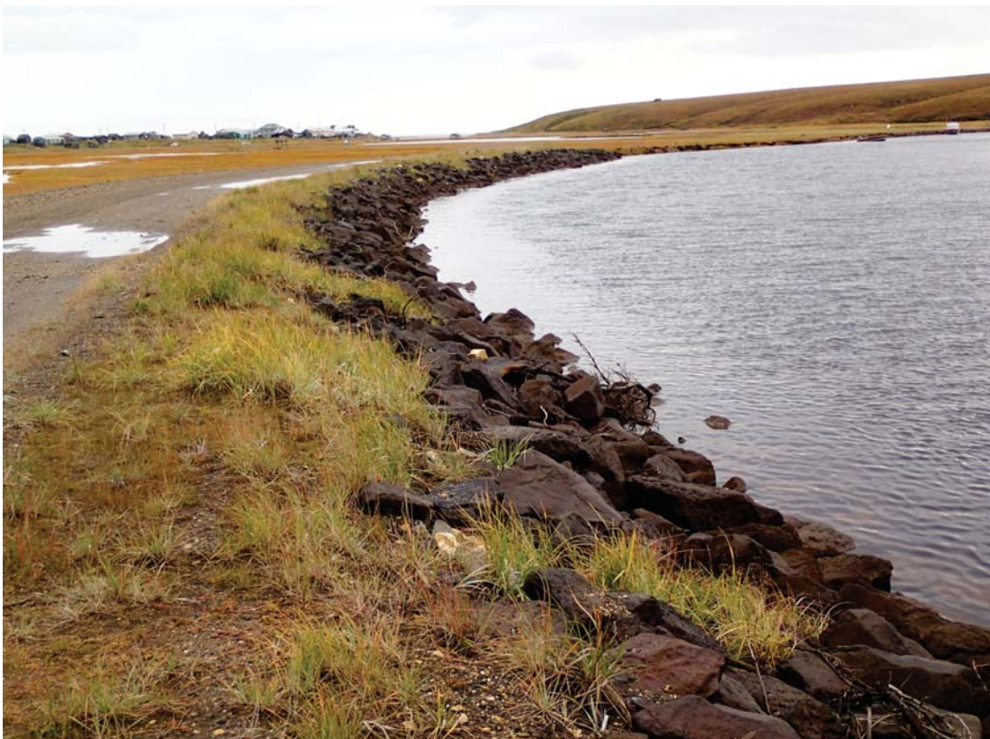
Looking downstream at the approximately 800-ft long revetment, September 2013
