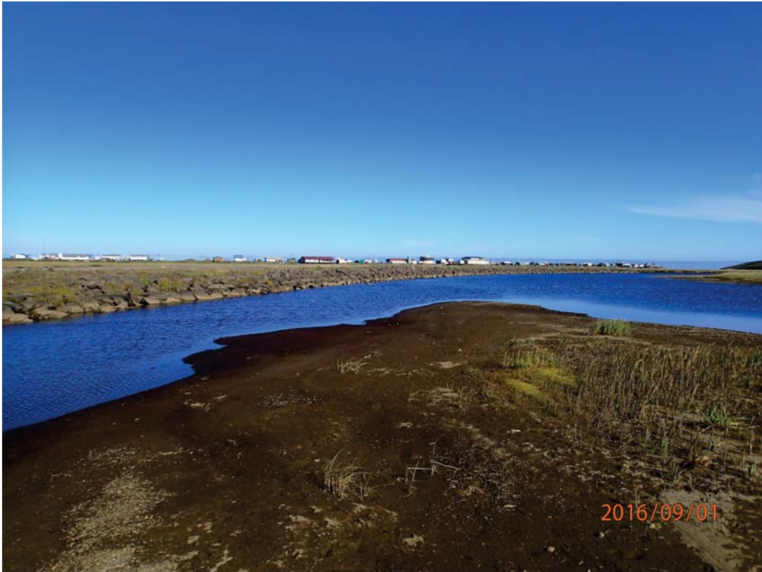
Looking at the revetment along the airport road, September 2016
