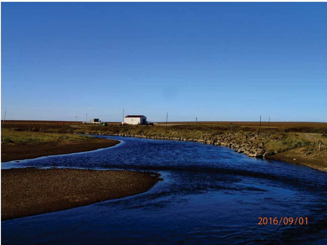
Revetment near the airport, September 2016
