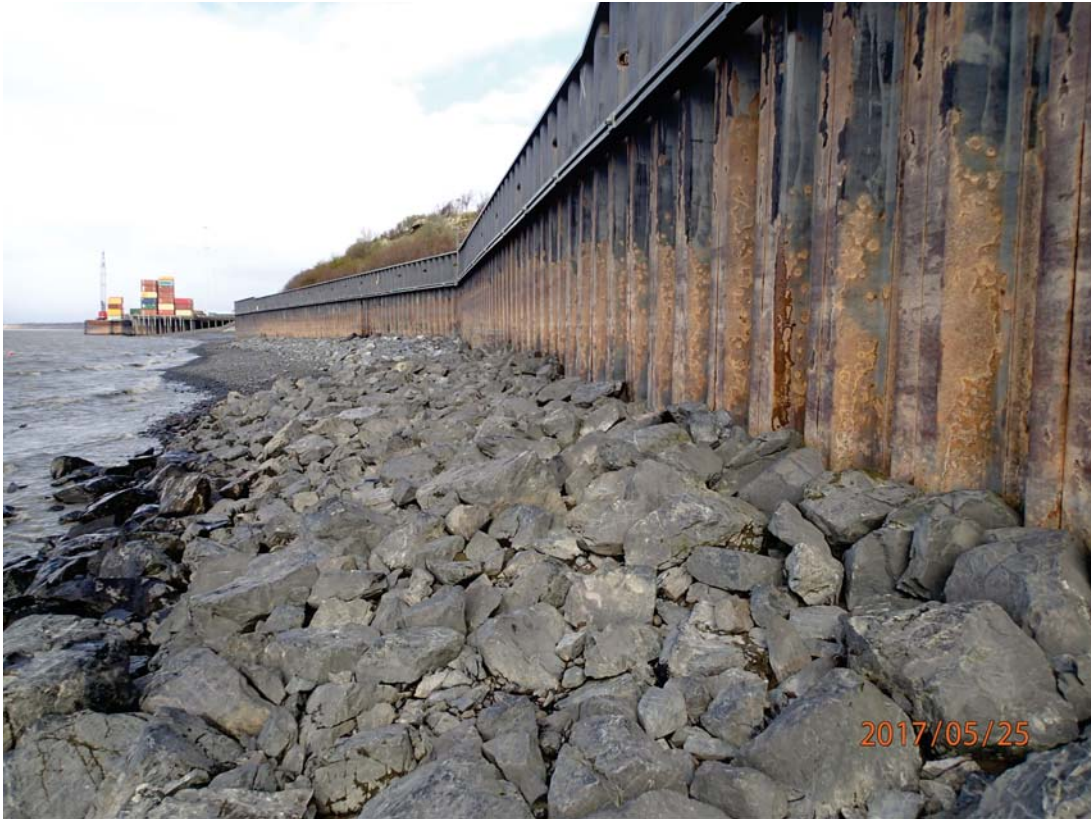
STA 21+00, Riprap @ Toe, Facing Downstream, May 2017
