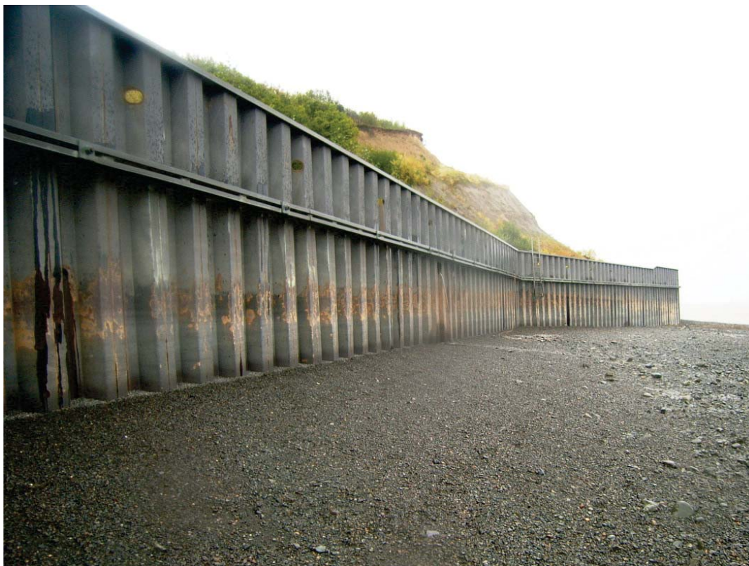
H-pile supported sheetpile bulkhead, September 2008
