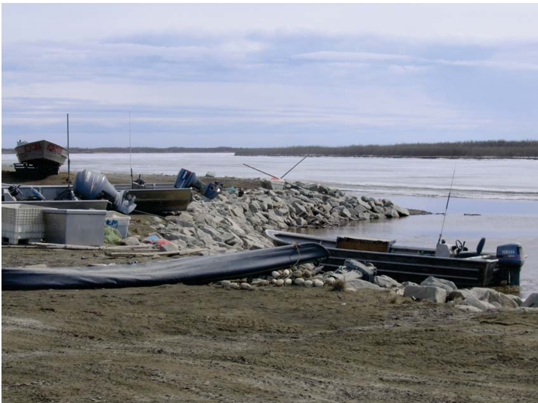
Emmonak streambank protection, 16 May 2007
