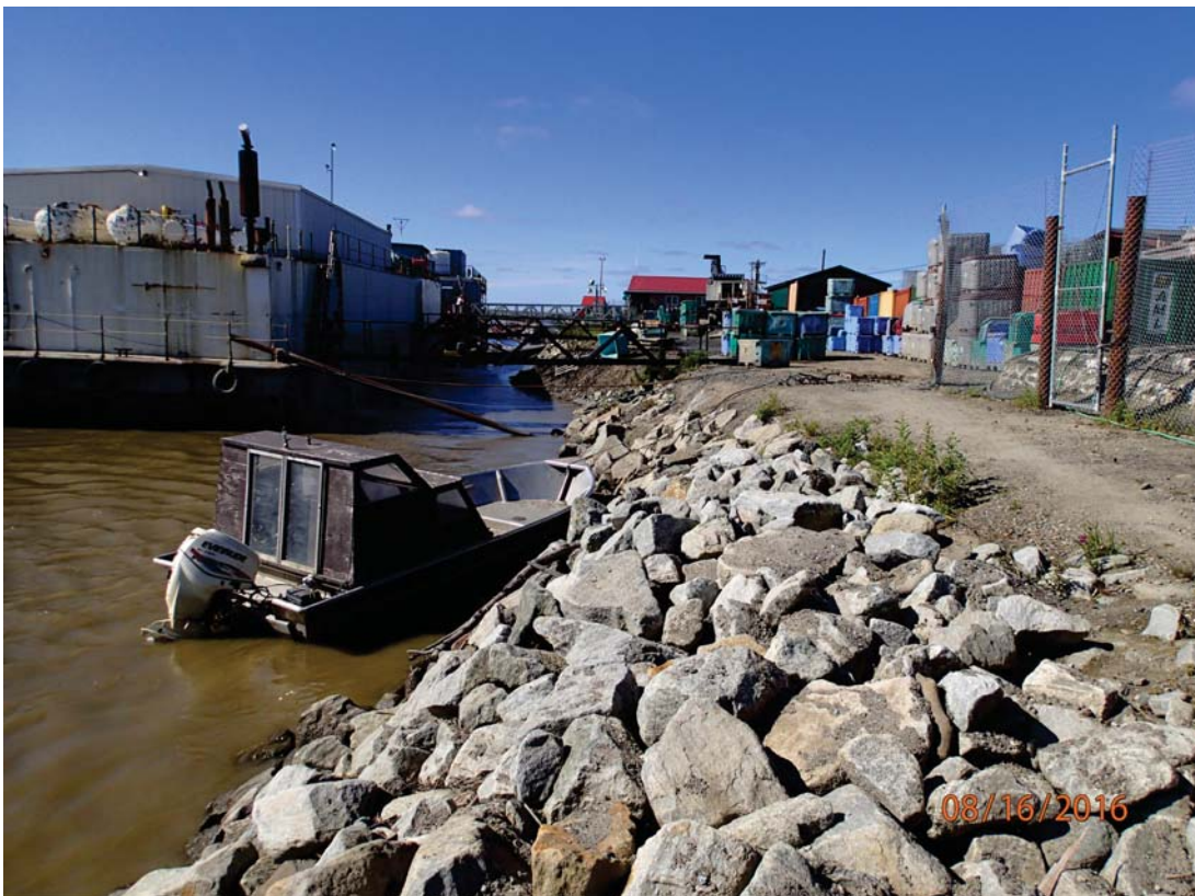
Emmonak revetment near fish processor, August 2016
