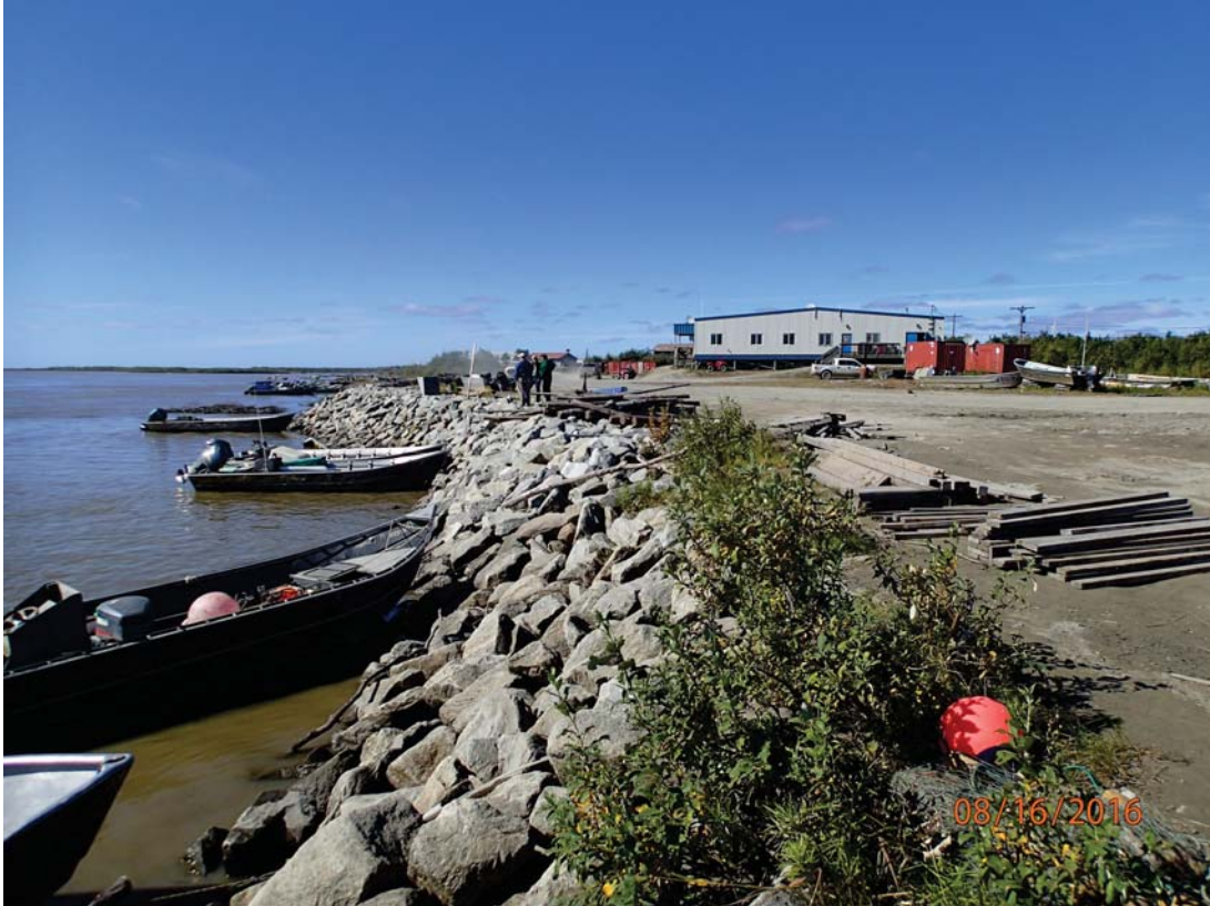
Emmonak revetment downstream of fish processor, August 2016
