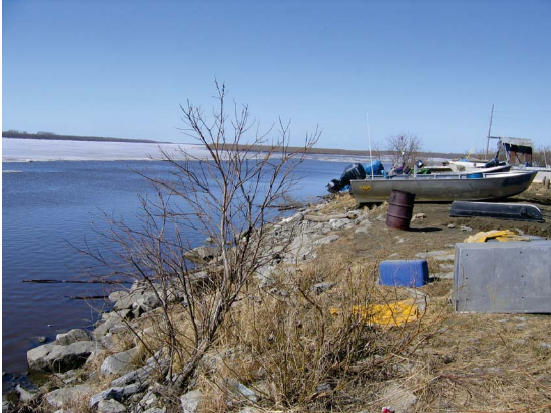
Emmonak streambank protection, 16 May 2007
