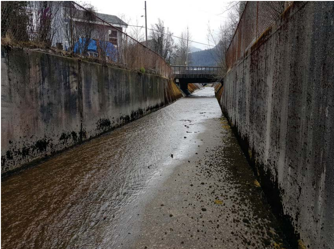
Concrete channel near 9th Street, 2017
