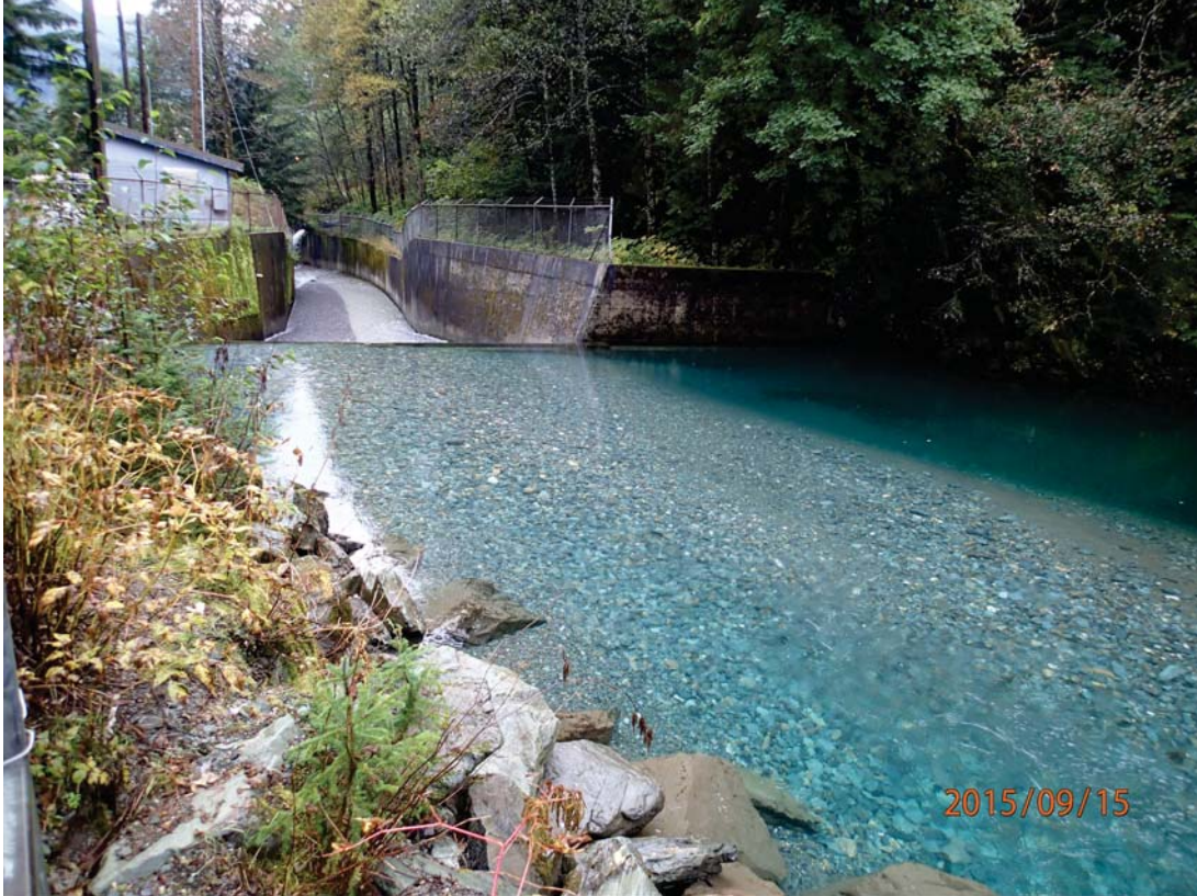
Weir and debris basin at upstream end of channel, September 2015
