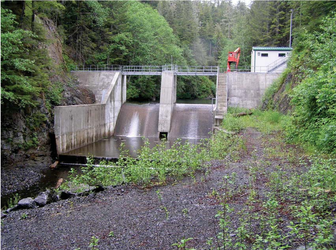
Downstream of Kake Dam, June 2010
