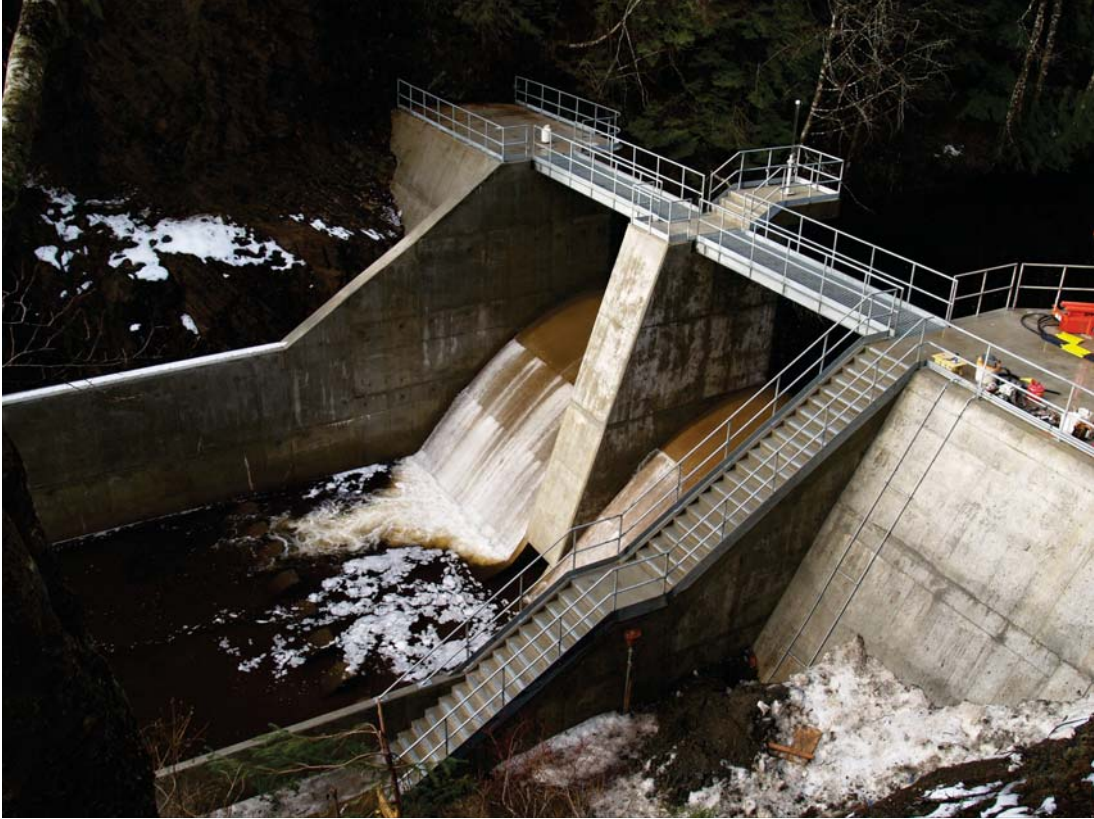
Downstream of Kake Dam during construction, January 2007
