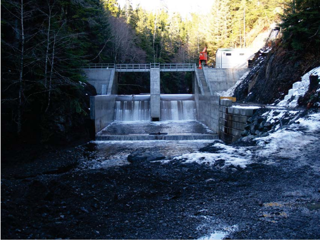
Downstream of Kake Dam during construction, January 2007
