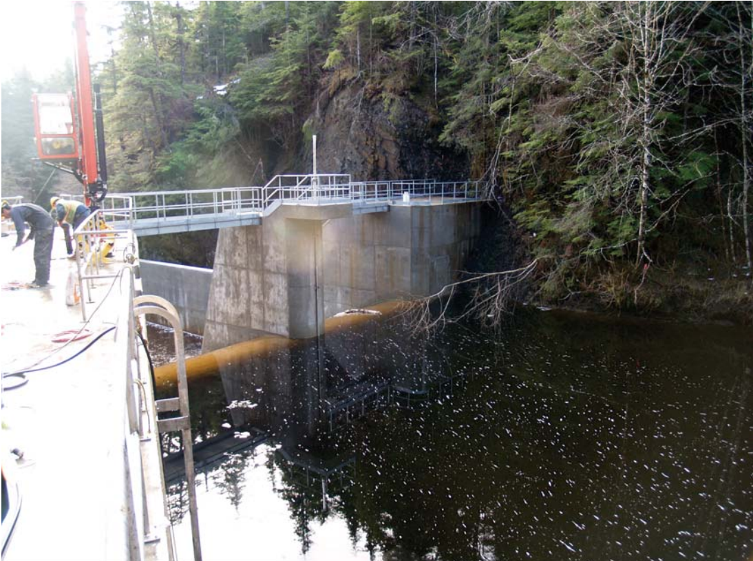
Upstream of Kake Dam during construction, January 2007
